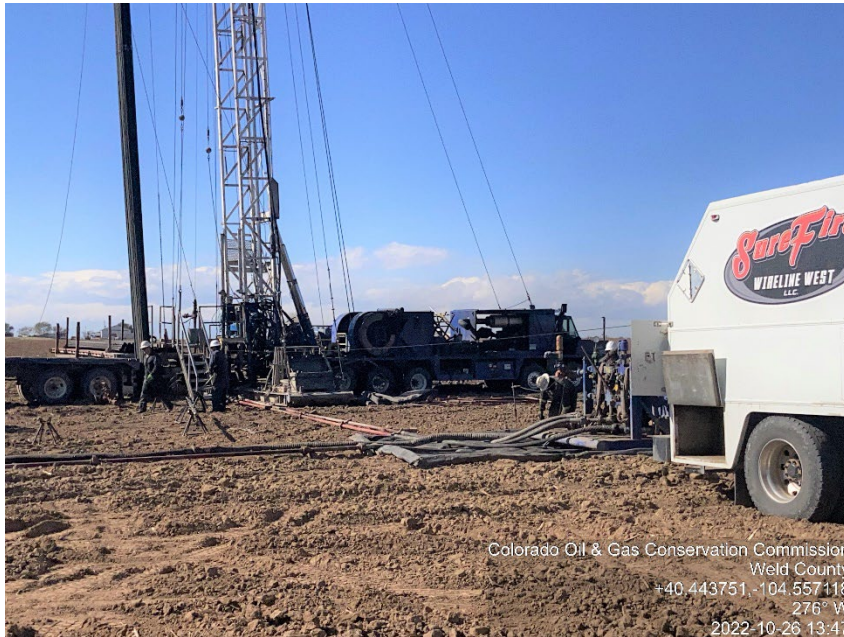
Photo #1 Noffsinger 22-33 (05-123-20237) Wellsite Plugged & Abandoned | PA Plugging Operations: Cementing | WK Initial plugs
