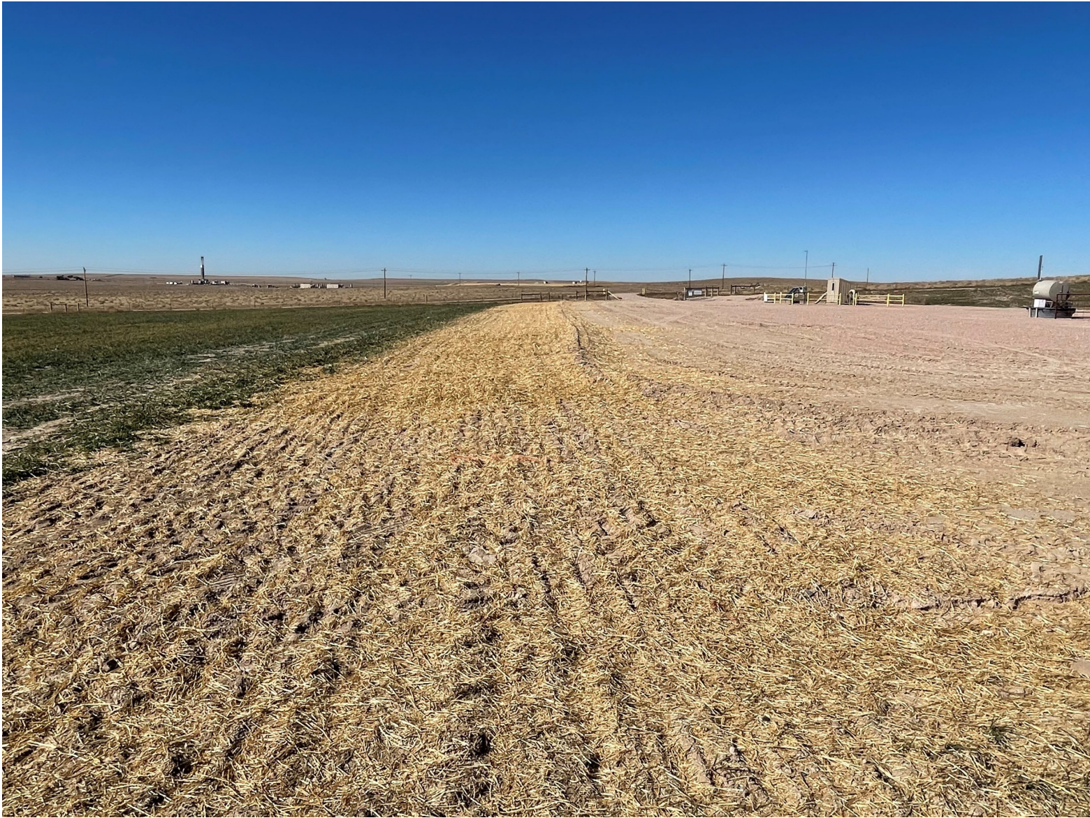
Dirt work completed to remove rill erosion and area has been reseeded and straw mulched. Standing off the southeast edge of pad looking west.
