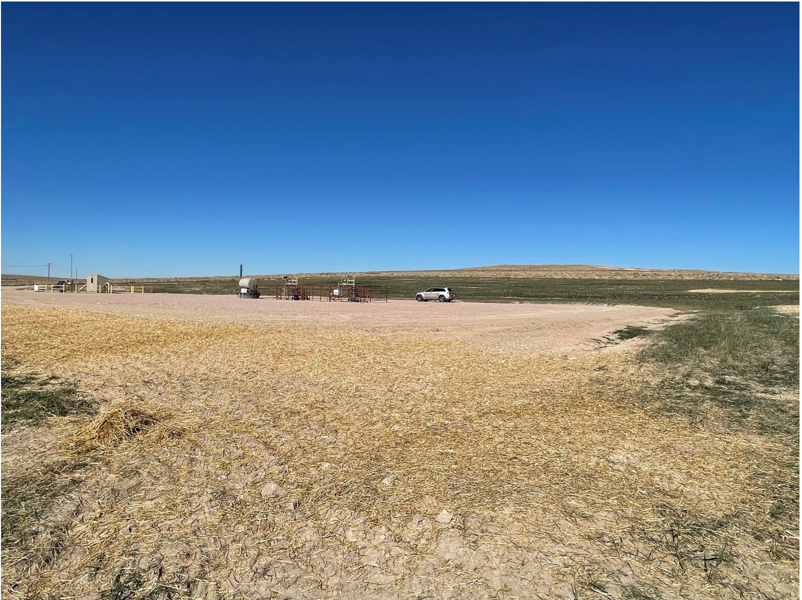
Sediment discharge cleaned up and area has been reseeded and straw mulched. Standing at the southeast corner looking northwest at the pad.
