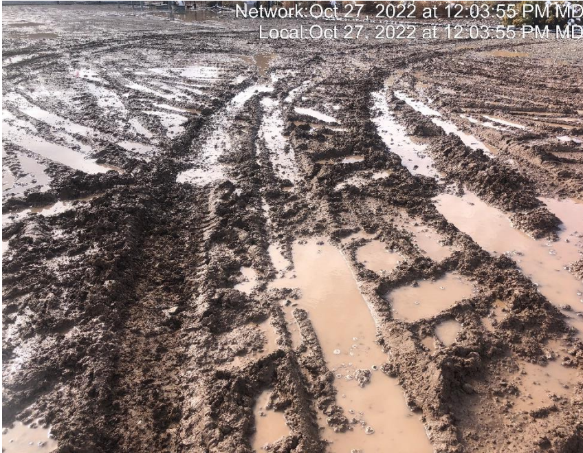
Photo #8192 Location lacks stabilization.
