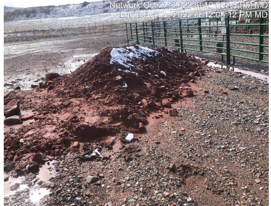
Photo #8196 BMP's have not been implemented around stockpiled soils.
