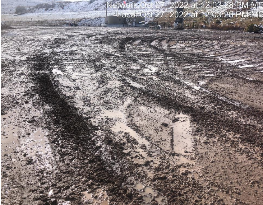
Photo #8190 Location lacks stabilization.
