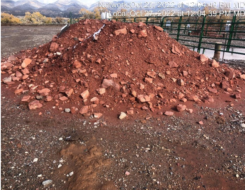
Photo #8194 BMP's have not been implemented around stockpiled soils.
