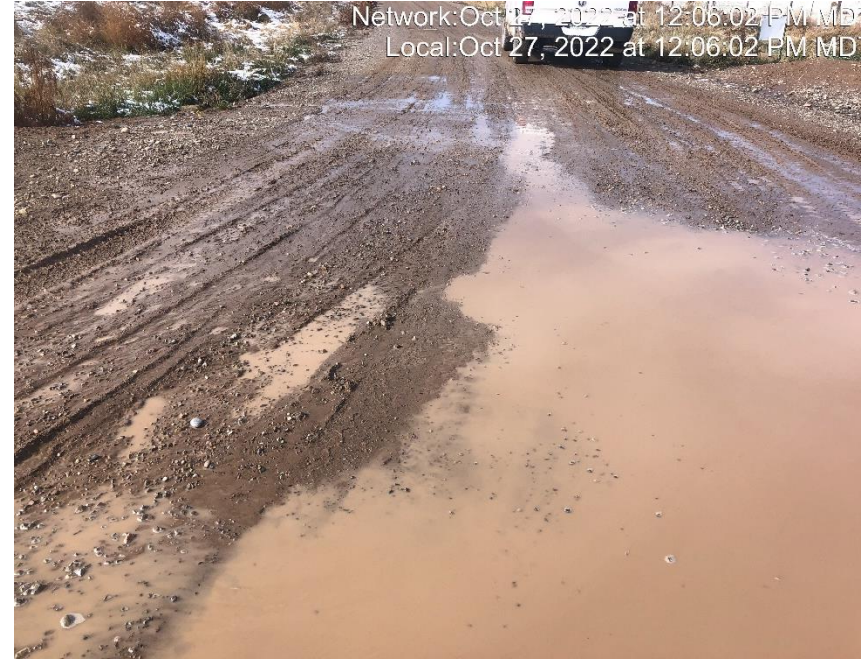
Photo #8198 Insufficient tracking BMP at entrance to location.
