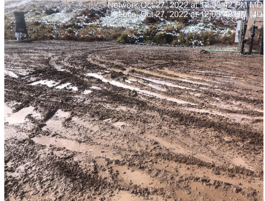
Photo #8191 Location lacks stabilization.
