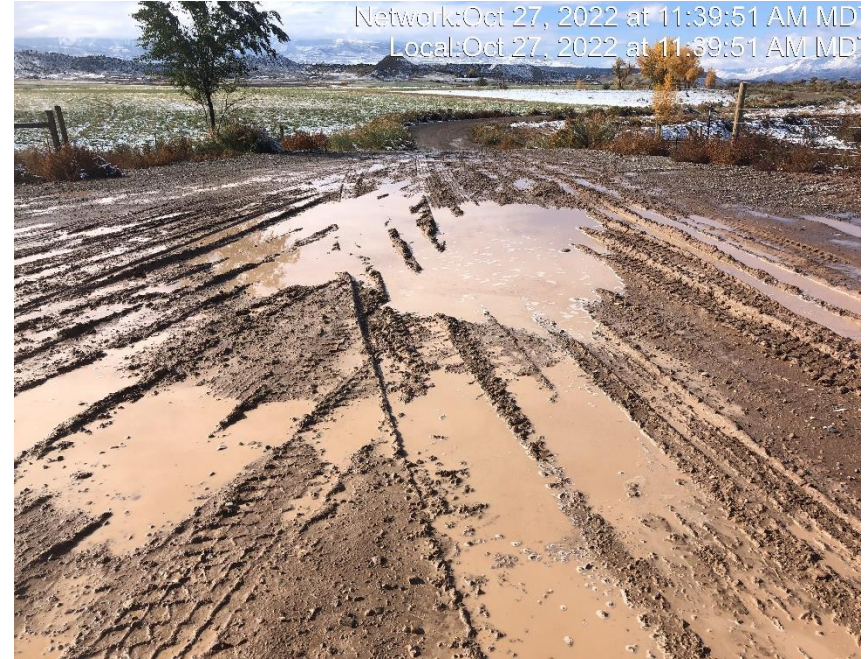
Photo #8187 Insufficient tracking BMP at entrance to location.
