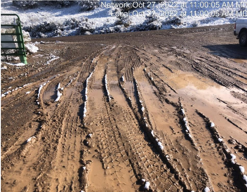
Photo #8177 Insufficient tracking BMP at entrance to location.
