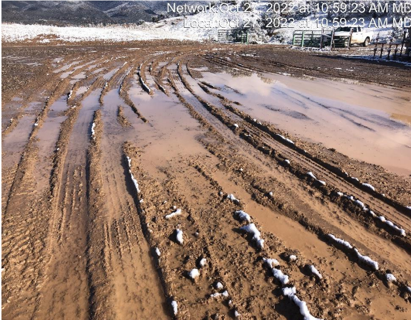
Photo #8175 Location lacks stabilization.
