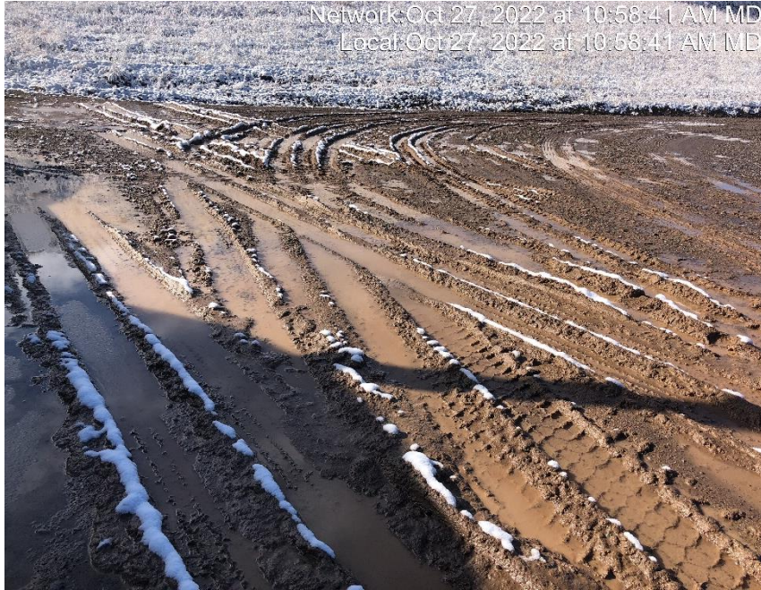
Photo #8172 Location lacks stabilization.
