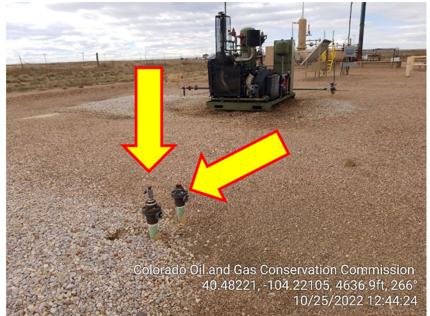
Photo 8 – Unmarked Risers
