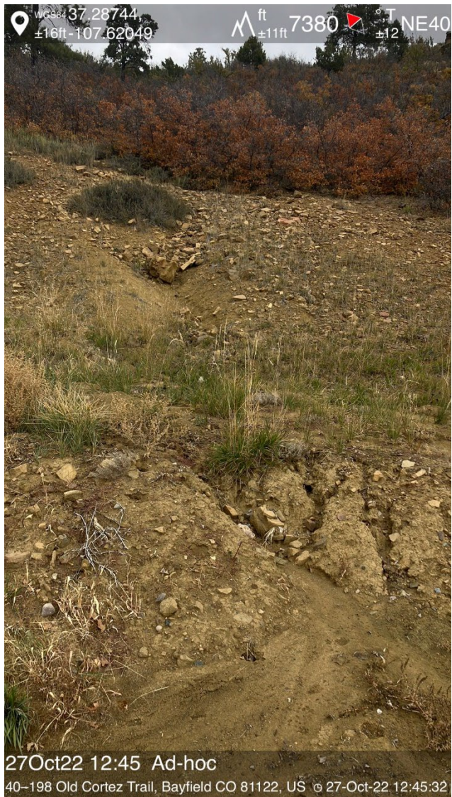
IMG 05 Erosion channel on cut slope
