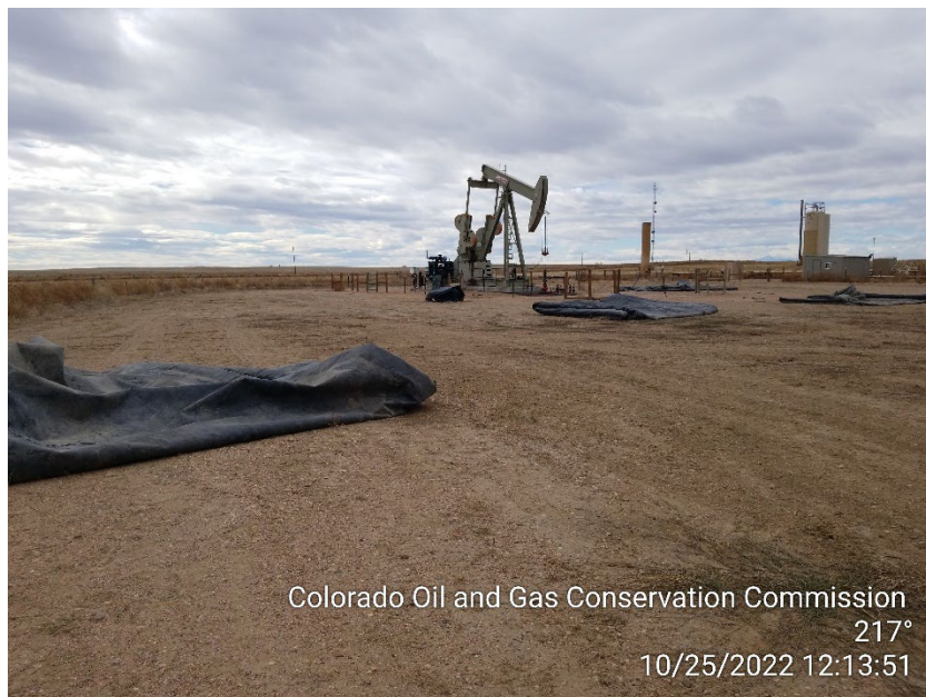
Photo 1 – Unused Secondary Containment on Location
