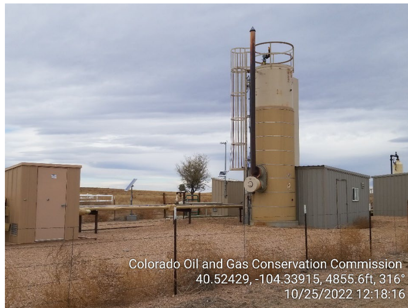
Photo 6 – Heater Treater
