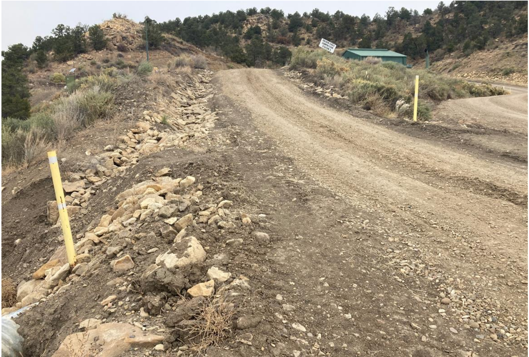
PHOTO 4: ROAD MATERIAL HAS ALSO BEEN ADDED TO THE LOCATION ACCESS AND IT HAS BEEN CROWNED TO ENCOURAGE SHEET FLOW AND DIRECT SURFACE RUN OFF TO THE ROCKED DIVERSION DITCH. THE CULVERT INLET HAS ALSO BEEN CLEANED AND RESET.
