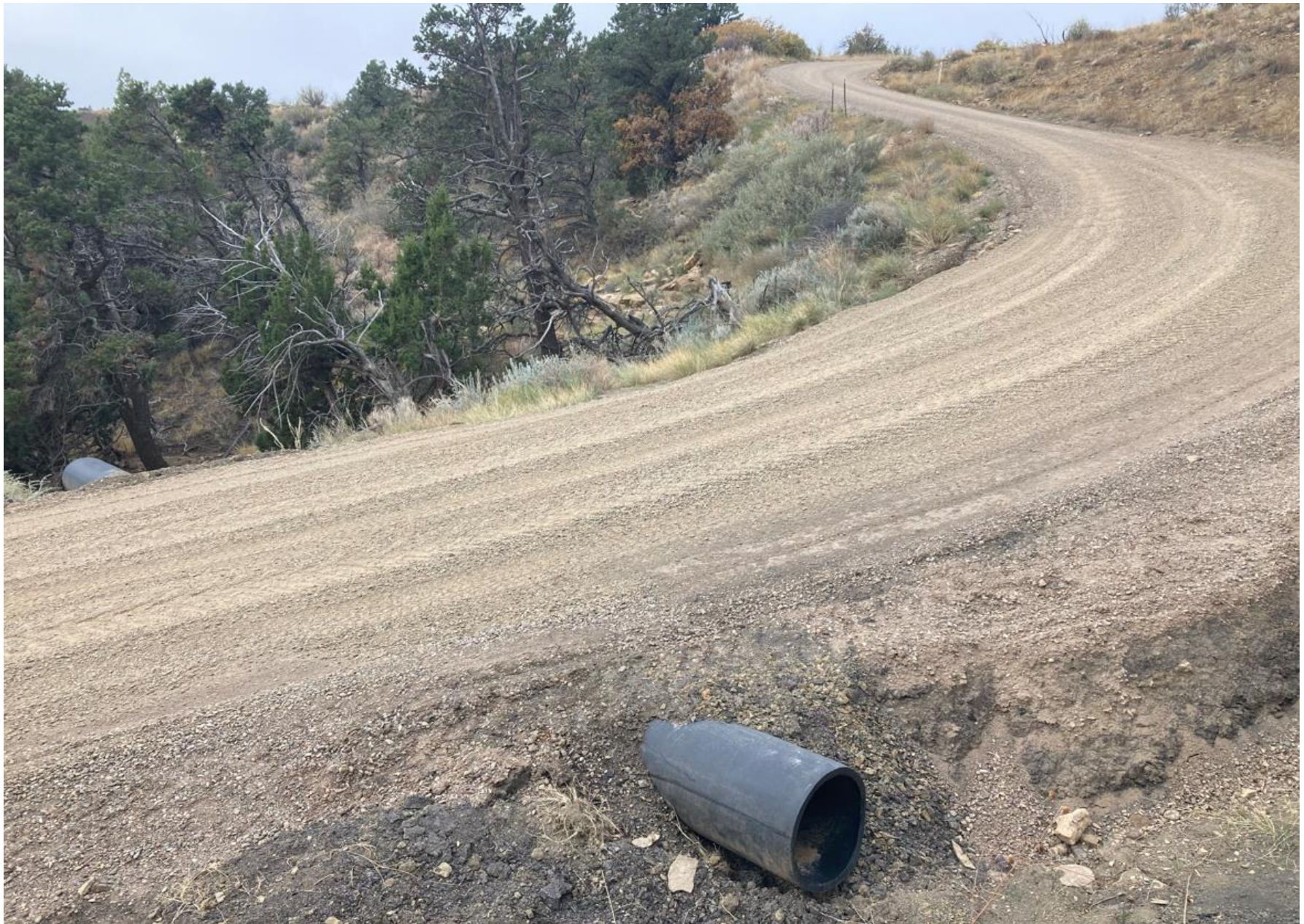
PHOTO 3: A CULVERT HAS BEEN ADDED ON THE MAIN ACCESS, CLIMBING ABOVE THE COMPRESSOR LOCATION. ROAD MATERIAL WAS ADDED ALONG THE MAIN ACCESS, THE ROAD SURFACE WAS CROWNED TO CREATE SHEET FLOW AND PROPERLY DIRECT SURFACE RUN OFF.
