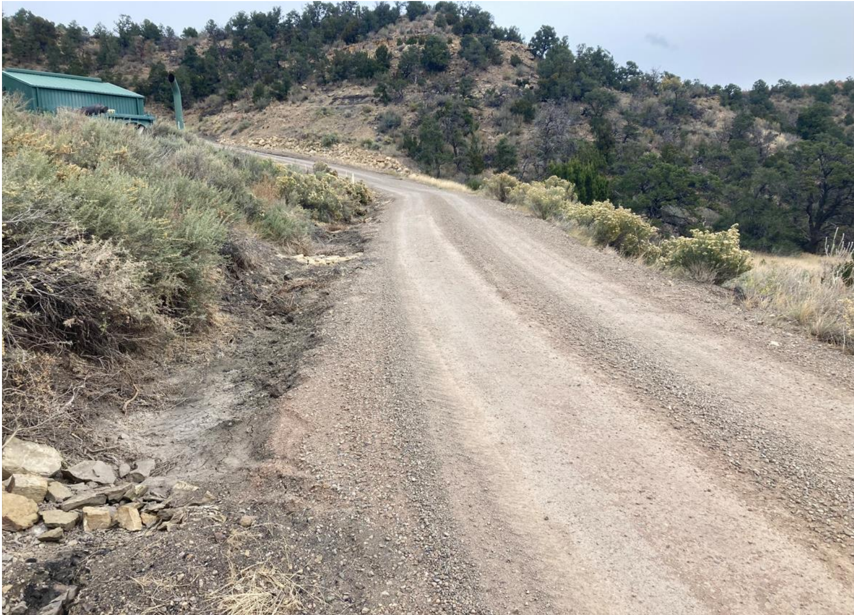
PHOTO 1 & 2: MAINTENANCE HAS BEEN PERFORMED TO THE ACCESS ROAD TO CORRECT ERROSION CHANELS AND VEHICLE RUTTING. THE DIVERSION DITCHES ALONG THE ROAD SIDE HAVE BEEN REDEFINED AND CHECK DAMS ADDED TO PROPERLY SLOW AND DIVERT STORMWATER.
