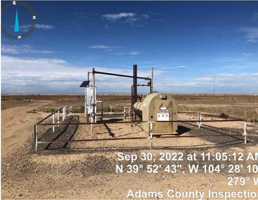
Photo#5 Separator/Gas Meter
