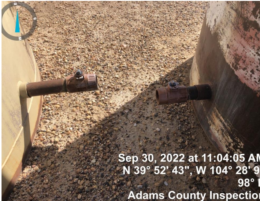
Photo#3 Corrective Action: Bull Plugs Missing
