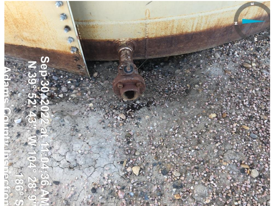
Photo#4 Corrective Action: Bull Plugs Missing
