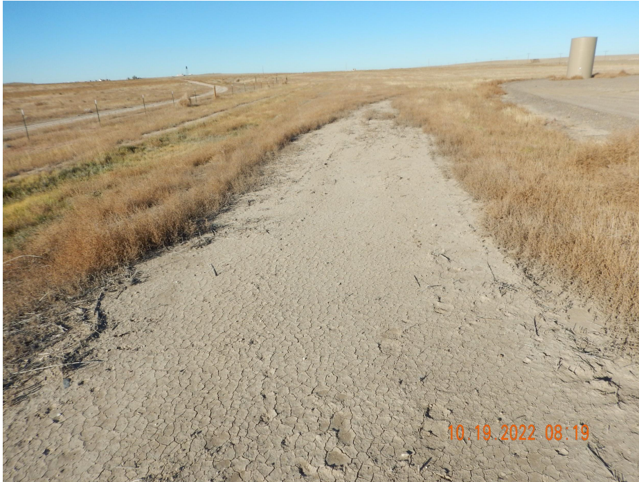
Photo 11. Photo taken from southeastern interim area, facing West. Photo illustrates what appears to be a potential topsoil stockpile lacking vegetative growth and is not stabilized.
