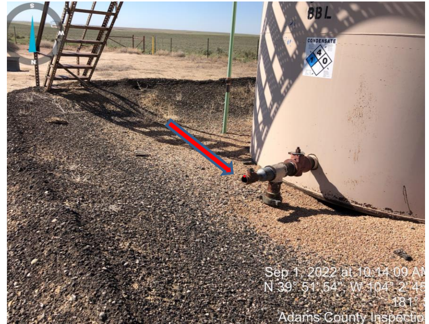
Photo #2 Tank missing bull plug.
