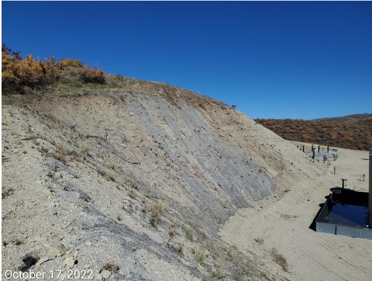
Photo 5: Photo taken from the cut slopes. Photo shows the erosion control blankets previously implemented have not been maintained in a proper functioning condition per good engineering practices. Erosion degradation has persisted.
