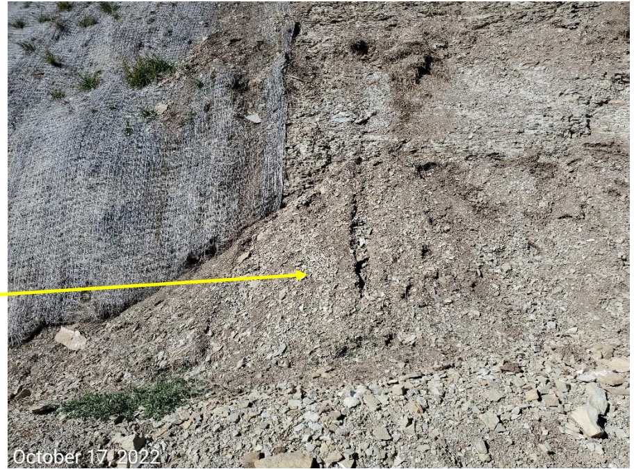
Photo 4: Photo taken from the toe of the cut slopes. Photo shows sediment deposition due to erosion degradation at the cut slopes.
