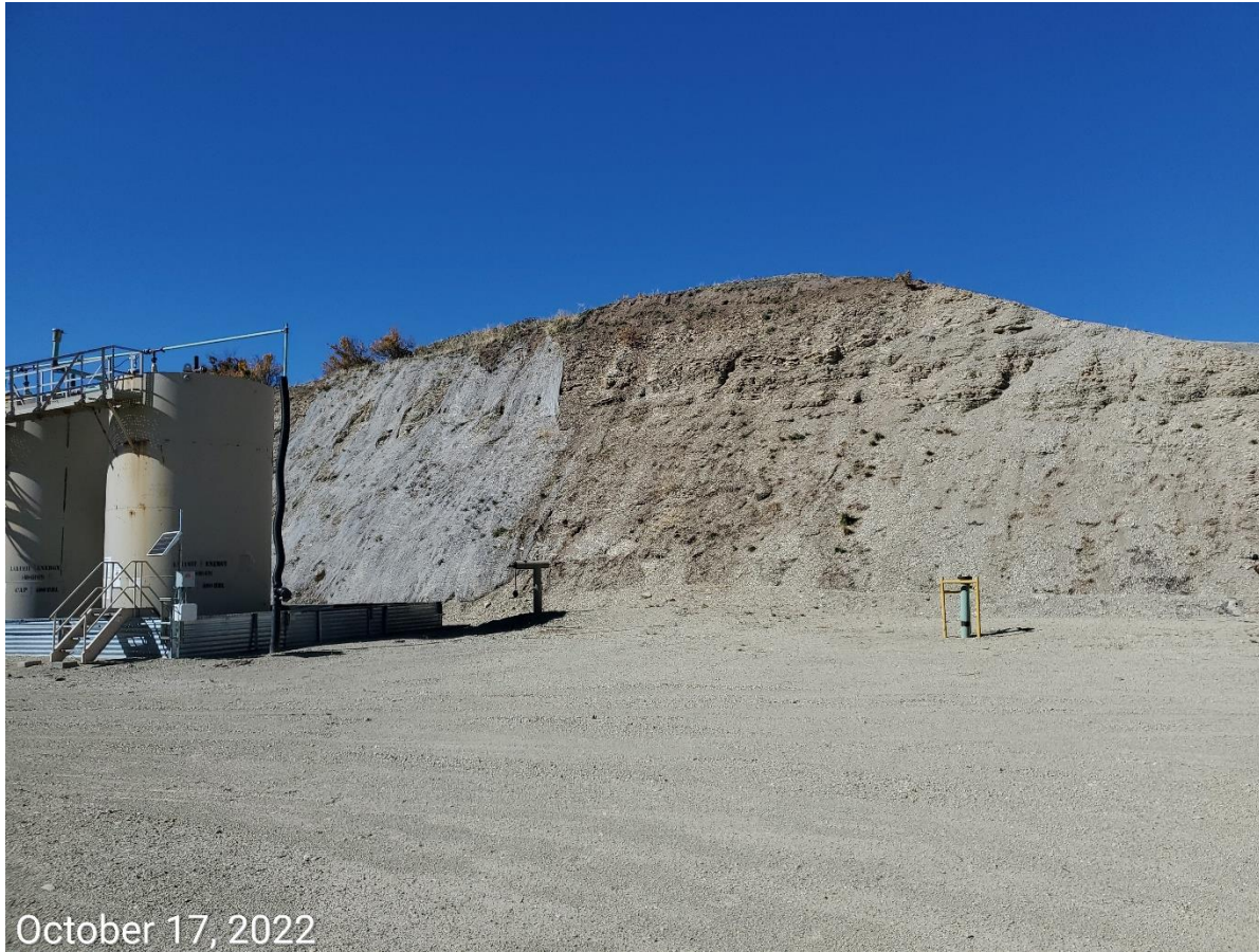
Photo 1: Photo taken from the Location, facing north. Photo shows large areas where control measures to protect, stabilize, as well as to minimize erosion and degradation at the cut slopes of the Location remain missing or insufficient.
