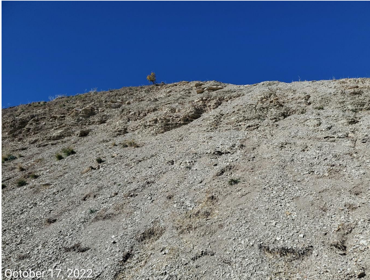
Photo 2: Photo shows large areas where control measures to measures to protect, stabilize, as well as to minimize erosion and degradation at the cut slopes of the Location remain missing or insufficient.
