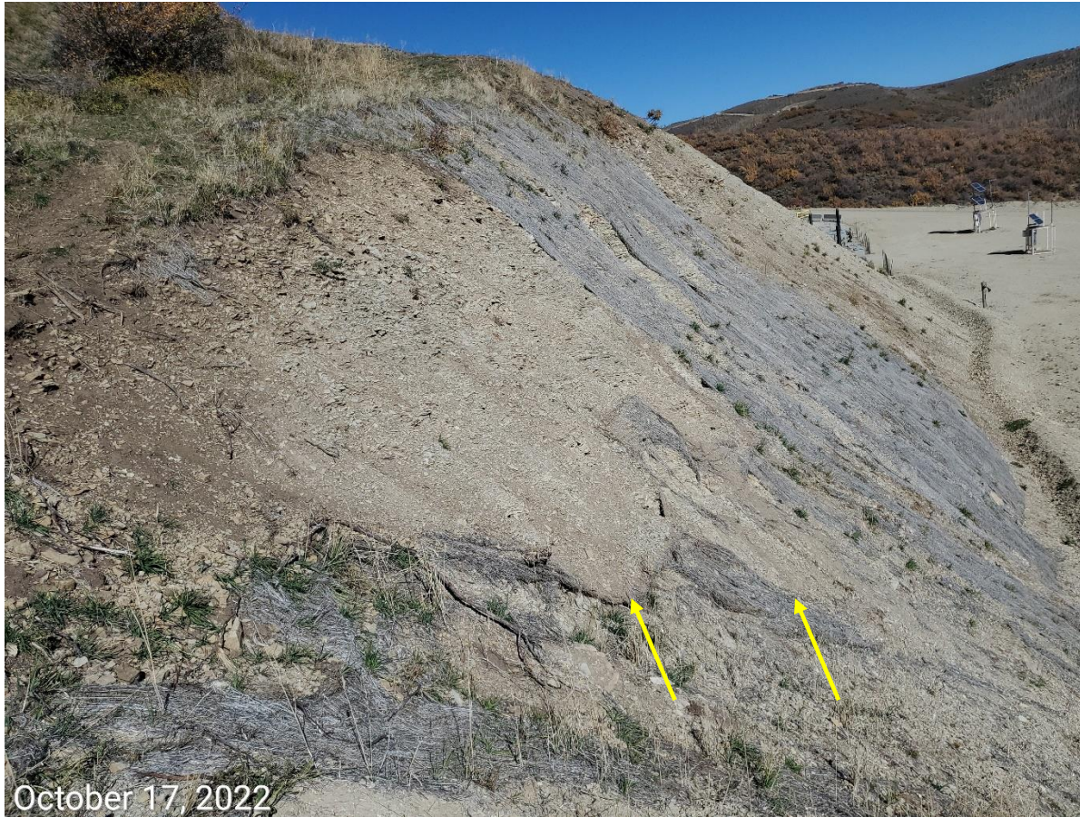
Photo 3: Photo taken from the cut slopes. Photo shows the erosion control blankets previously implemented have not been maintained in a proper functioning condition per good engineering practices. Erosion degradation has persisted. Arrow shows blanket in disrepair, as well as sediment/material eroding from the slopes covering remaining erosion blankets.
