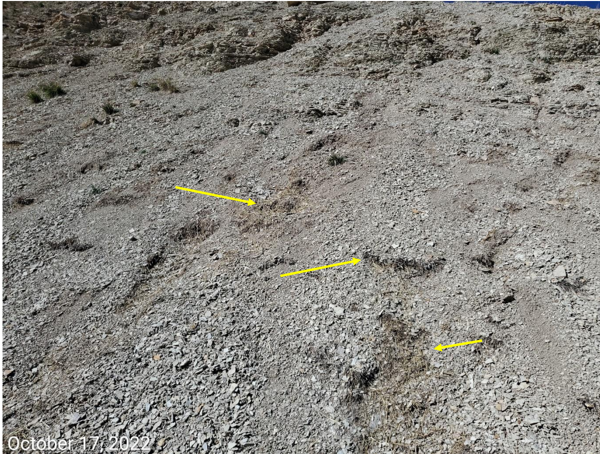
Photo 3: Continued from photo 2. Photo shows sediment/material eroding from the slopes have covered what appears to have be straw mulch applied to the slopes. BMP observed inadequate to protect, stabilize, as well as to minimize erosion and degradation at the cut slopes; erosion degradation has persisted.
