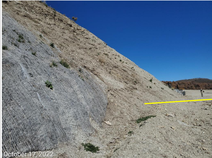
Photo 4: Photo taken from the toe of the cut slopes. Photo shows sediment deposition due to erosion degradation at the cut slopes.
