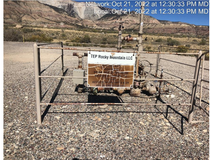
Photo #8141 Wellhead sign weathered and not legible.
