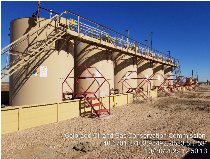
Photo 1 – Tank Battery
