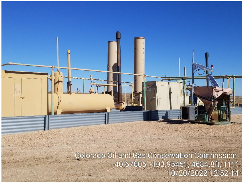
Photo 3 – Separators and ECDs
