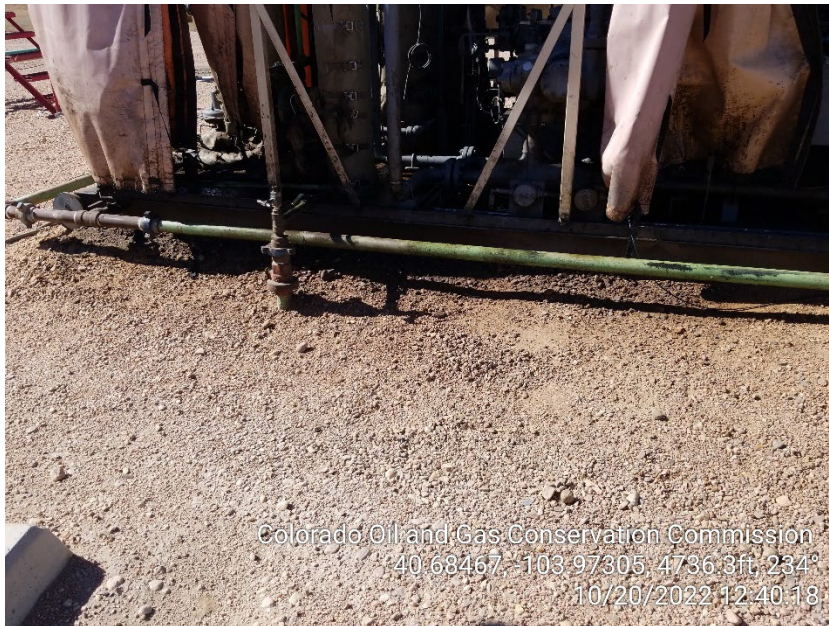
Photo 5 – Stained Soil at Compressor
