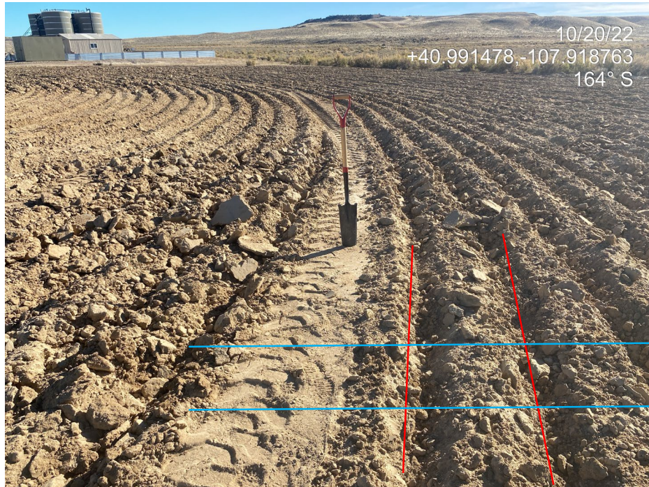
Photo 6. Photo shows a the Location has been ripped in one direction. Shovel was unable to penetrate a continuous strip of unripped soil. “Cross-ripping” means passes should be overlapping. Red line indicates direction of rip. Blue line indicates additional rip direction needed.
