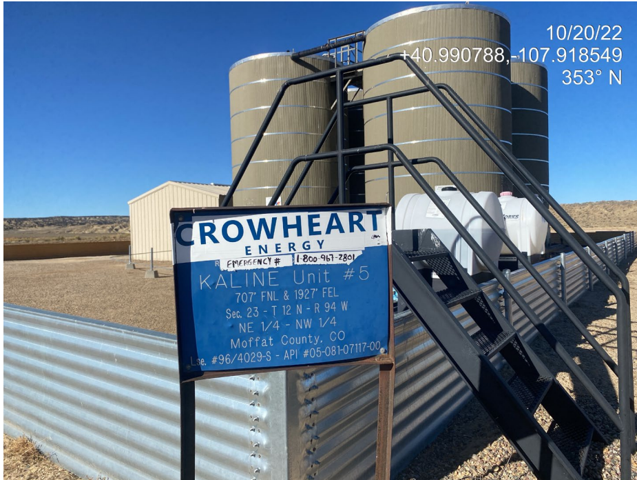
Photo 3. Photo shows the tank battery sign. Sign does not comply with Rule 605; Telephone number for local emergency services (911 where available) and the public road used to access the tank battery site are not posted.
