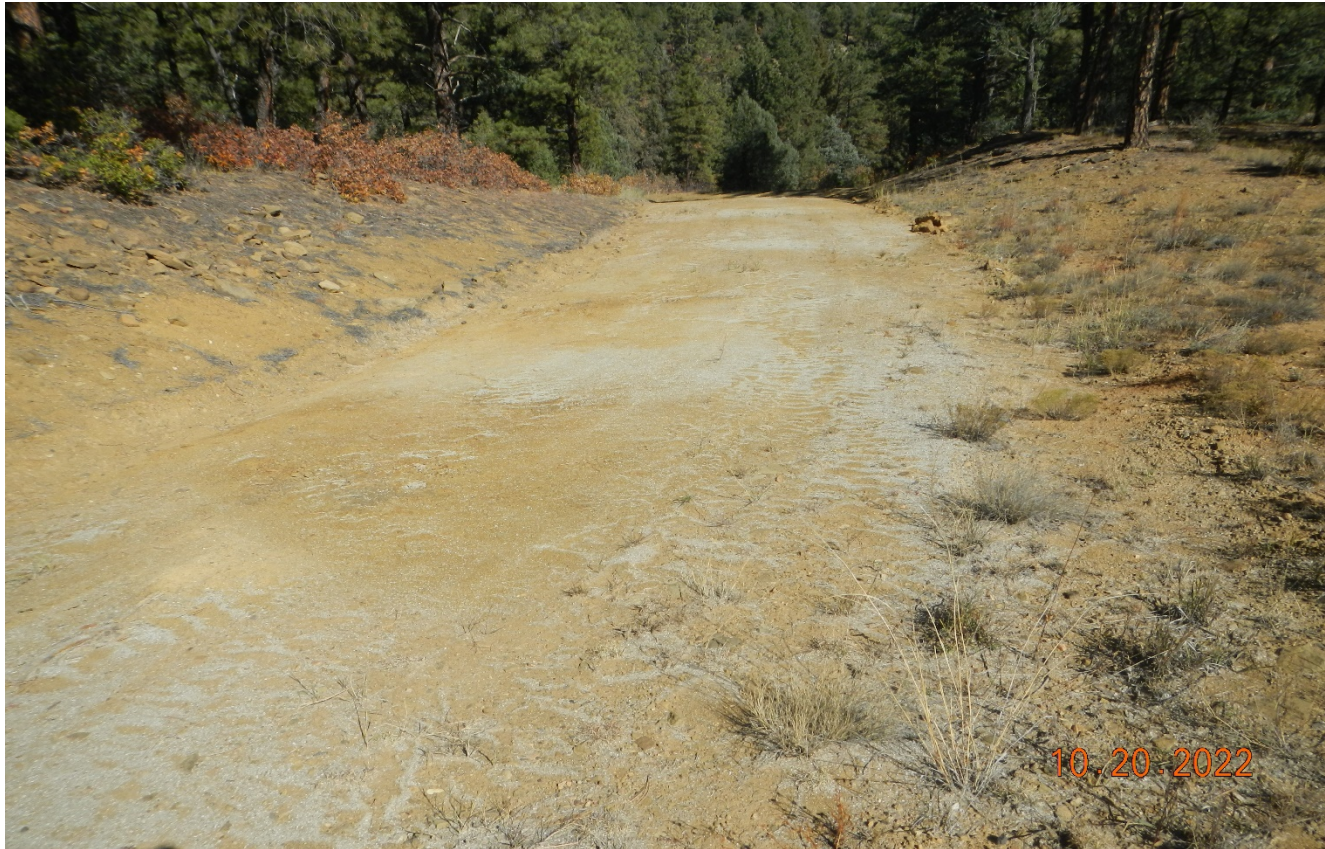
Photo 2. Facing northeast along the access road. The road has been regraded and repaired.
