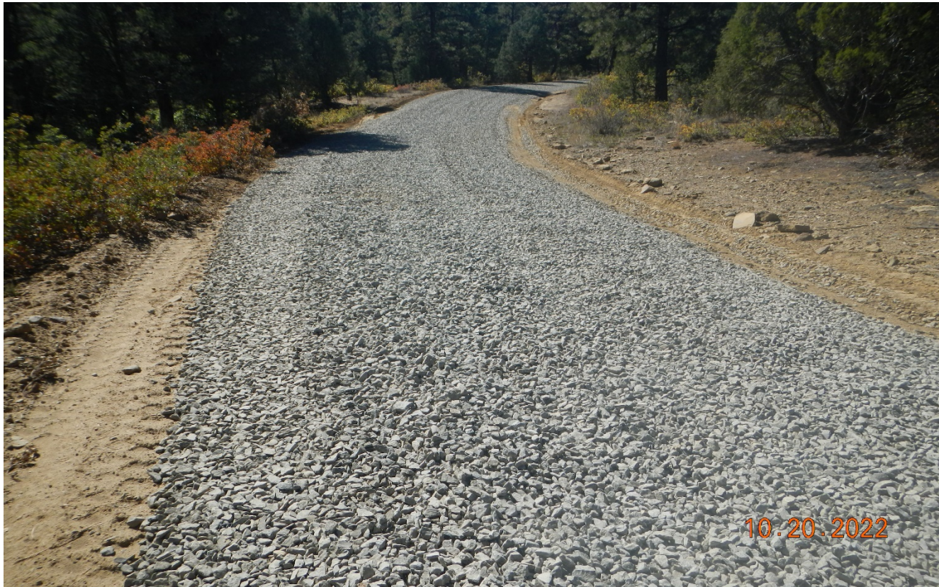
Photo 1. Facing south along the access road. This area of the road has been repaired and stabilized with gravel.
