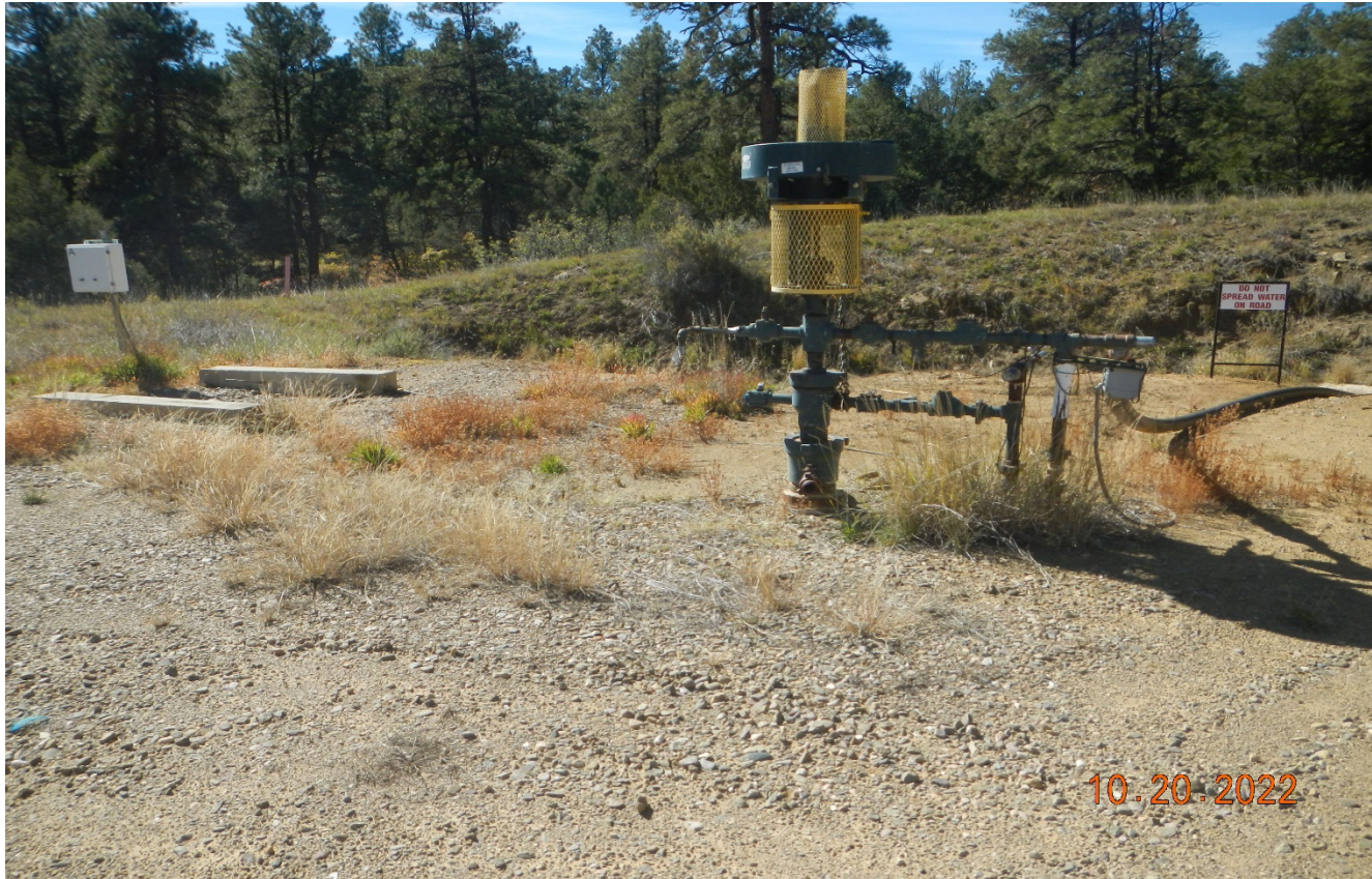
Photo 4. Facing toward the wellhead.
