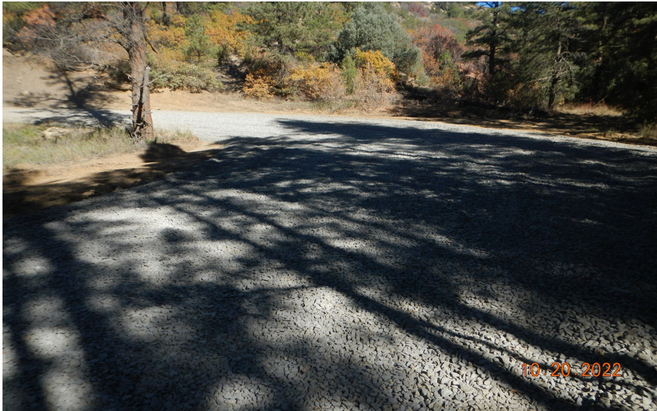
Photo 1. Facing south along the access road. This area of the road has been repaired and stabilized with gravel. Approximate Lat/Long:37.23652,-104.69804
