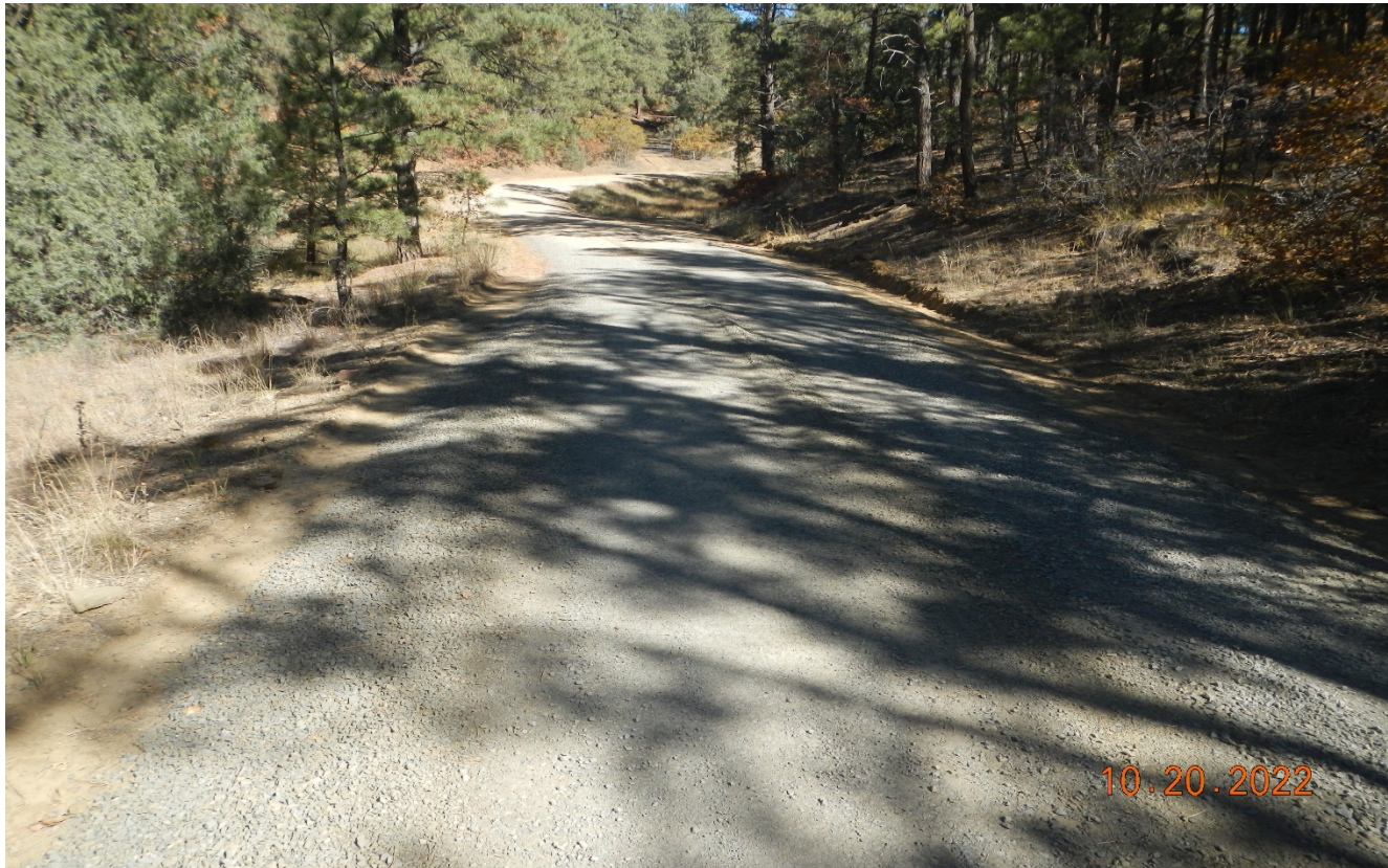
Photo 3. The road has been stabilized with gravel. Approximate Lat/Long:37.246320,-104.679854
