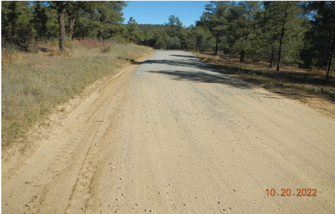
Photo 2. Facing south along the access road. This area of the road has been repaired and stabilized with gravel. Approximate Lat/Long:37.24515,-104.68856
