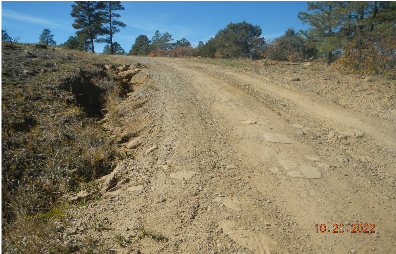
Photo 2. Facing west along the main access road. There is erosion along the roadside in this area. Previous corrective action was not completed.
