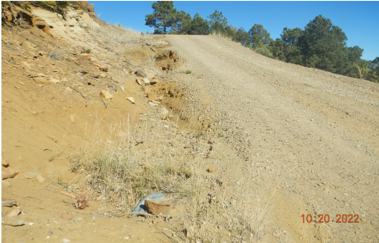
Photo 1. Facing northeast along the main access road past the compressor. There is erosion along the roadside in this area and the culvert is partially filled in with sediment. Previous corrective action was not completed.
