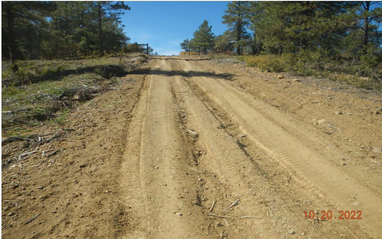
Photo 3. There is erosion and vehicle rutting along the access road near the location.
