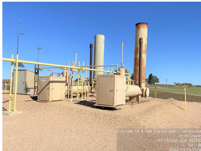
Photo #4 WPF III A18-2 Battery site Inactive / Shut-down ECDs, Separator
