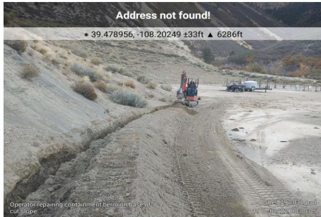
Operator Repairing Earthen Berm Identified in Photo #6
