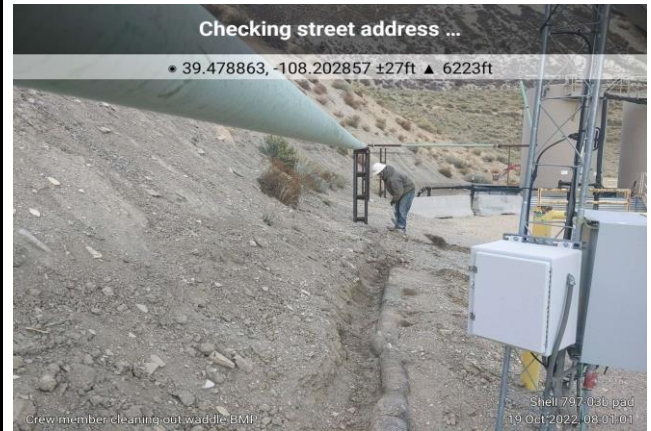
Maintaining Inundated Excelsior Wattle Identified in Photo #5
