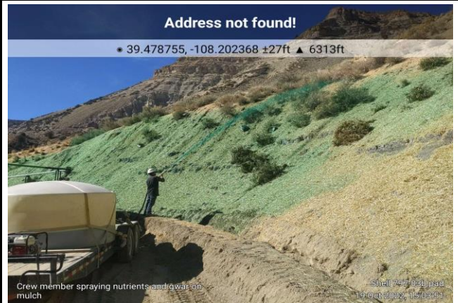
Applying Liquid Amenities/Tackifier
