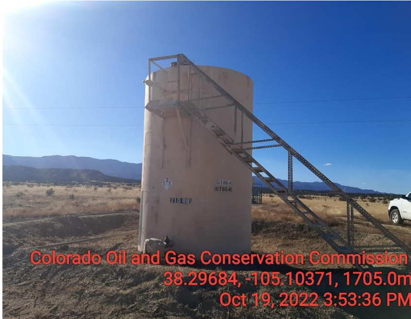
Photo 1 Unused equipment tank is not connected to anything
