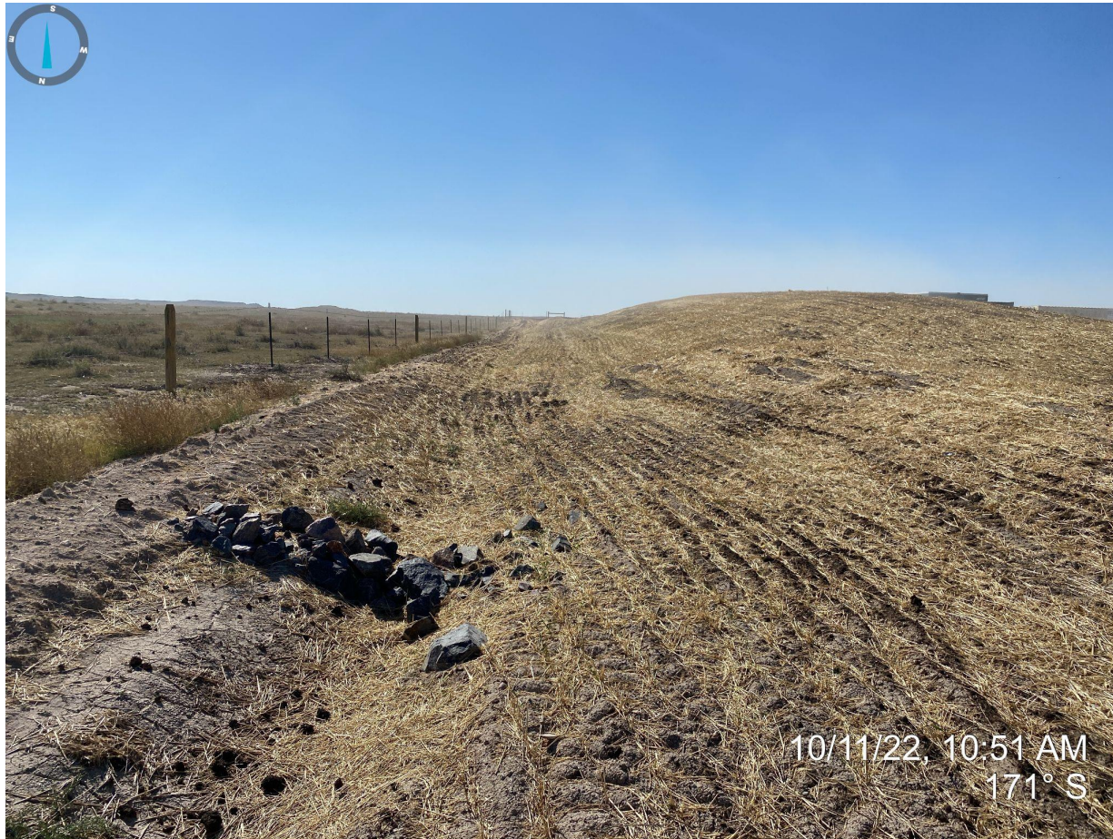
Photo 14. Taken from northeast portion near stockpile, facing south. Photo depicts topsoil stockpile has been stabilized with evidence of straw crimped into drill rows.
