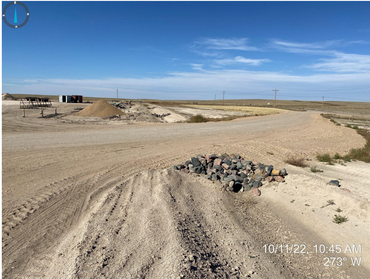
Photo 3. Taken near access road/location transition, facing west. Photo depicts rip-rap installed at inlet and outlet of culvert.
