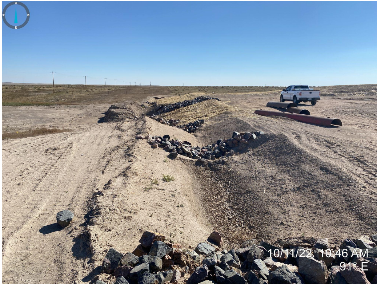
Photo 4. Taken near culvert, facing east. Photo depicts rip-rap has been installed in ditch.
