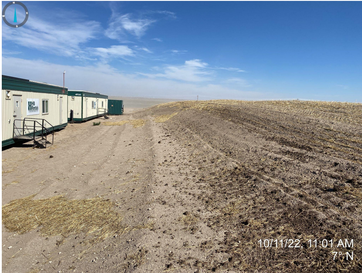
Photo 15. Taken near topsoil stockpile, facing north. Photo depicts western portion of stockpile is not stabilized and is susceptible to wind and water erosion.
