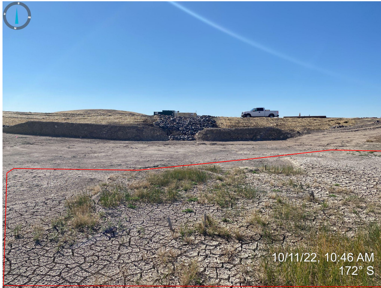
Photo 10. Taken north of detention area, facing south. Photo depicts deposited sediment that left detention area, identified in previous inspection.
