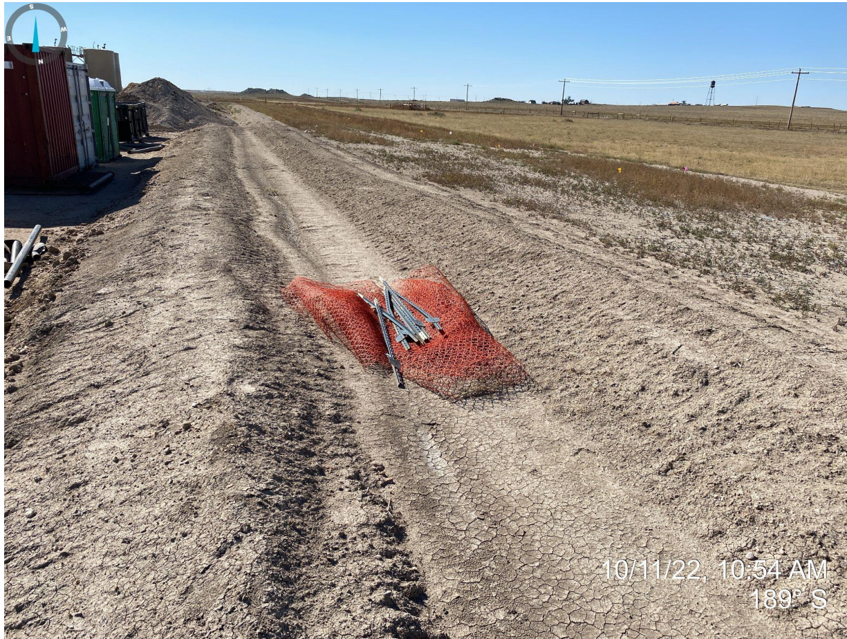
Photo 22. Taken from western portion of location, facing south. Fencing material observed in ditch and berm BMP.
