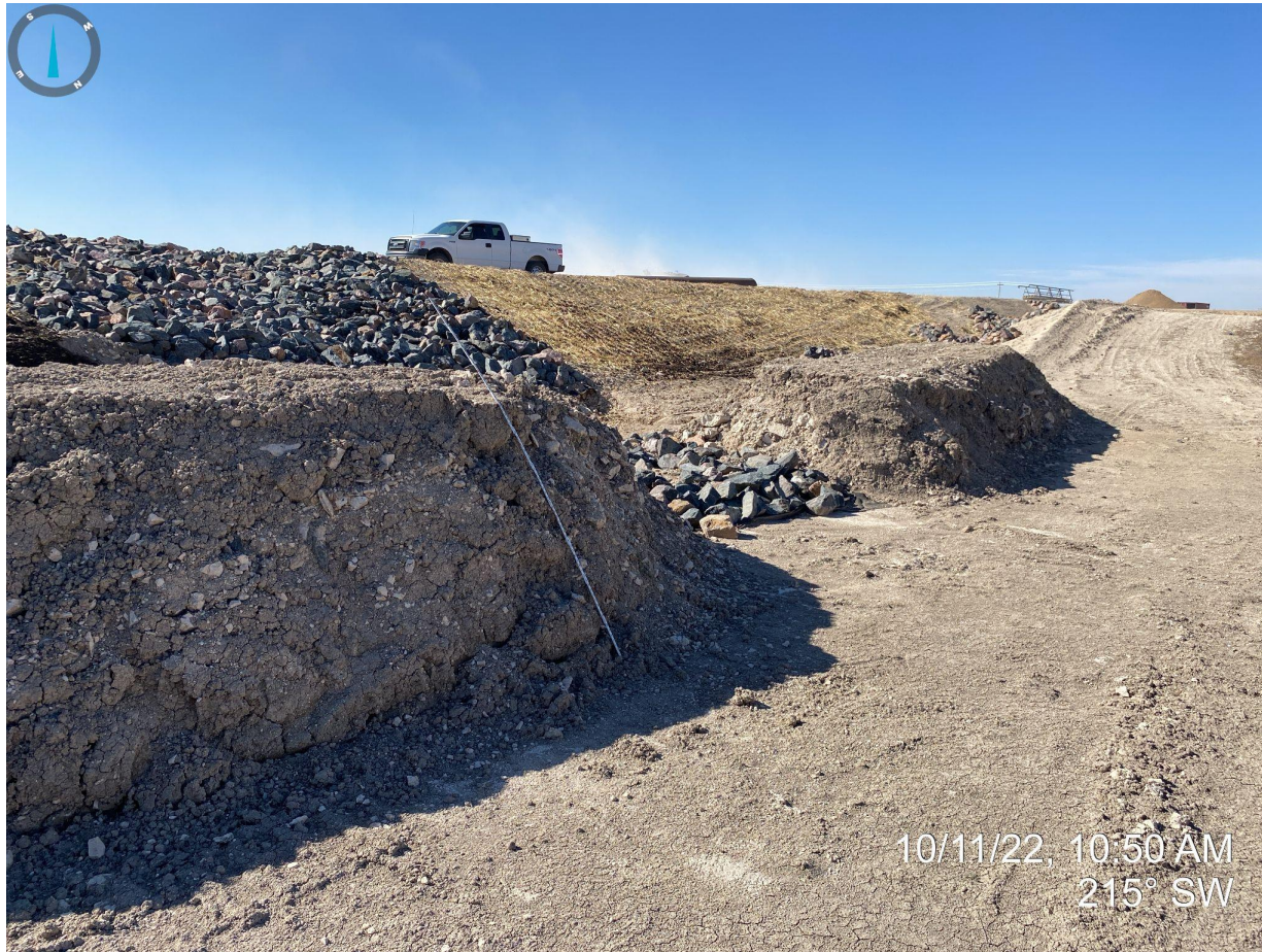
Photo 9. Taken north of detention area, facing west. Photo depicts unconsolidated material in berms; north walls of the berms appear vertical. 6.5' measuring stick for scale.
