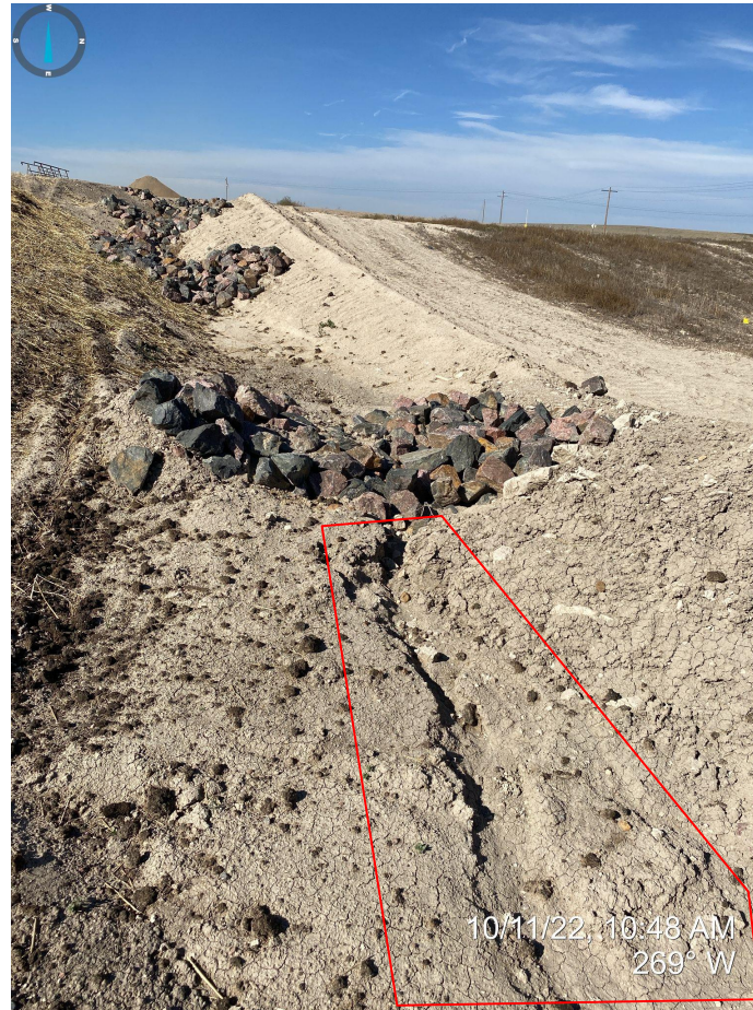
Photo 5. Taken from detention area, facing west. Photo depicts rill erosion in ditch, outlined in red.
