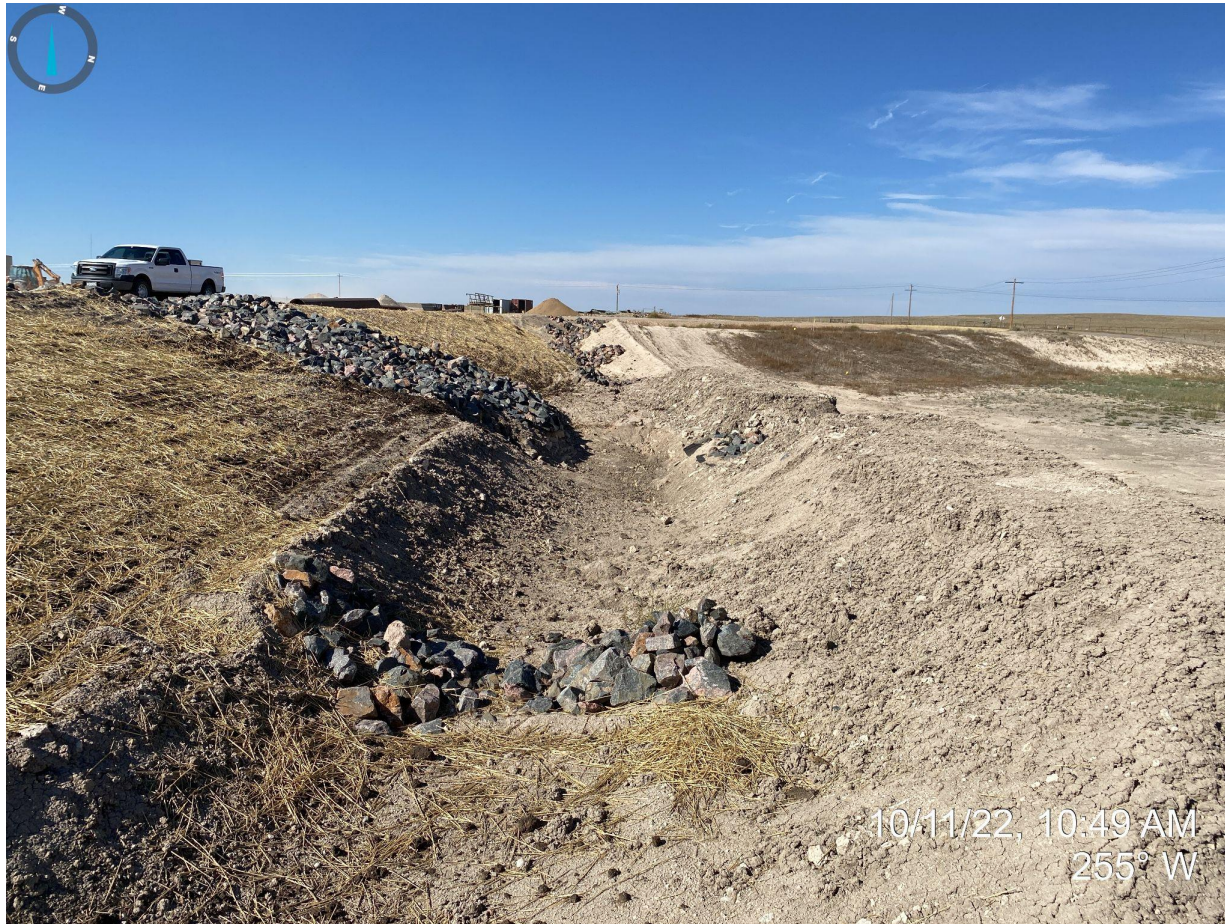
Photo 6. Taken east of detention area, facing west. Photo depicts rip-rap installed around inflows of BMPs.
