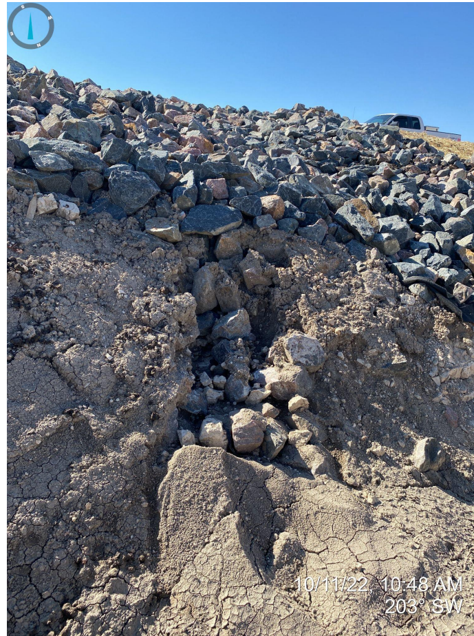
Photo 8. Close-up photo of rill erosion on inflow rip-rap area.
