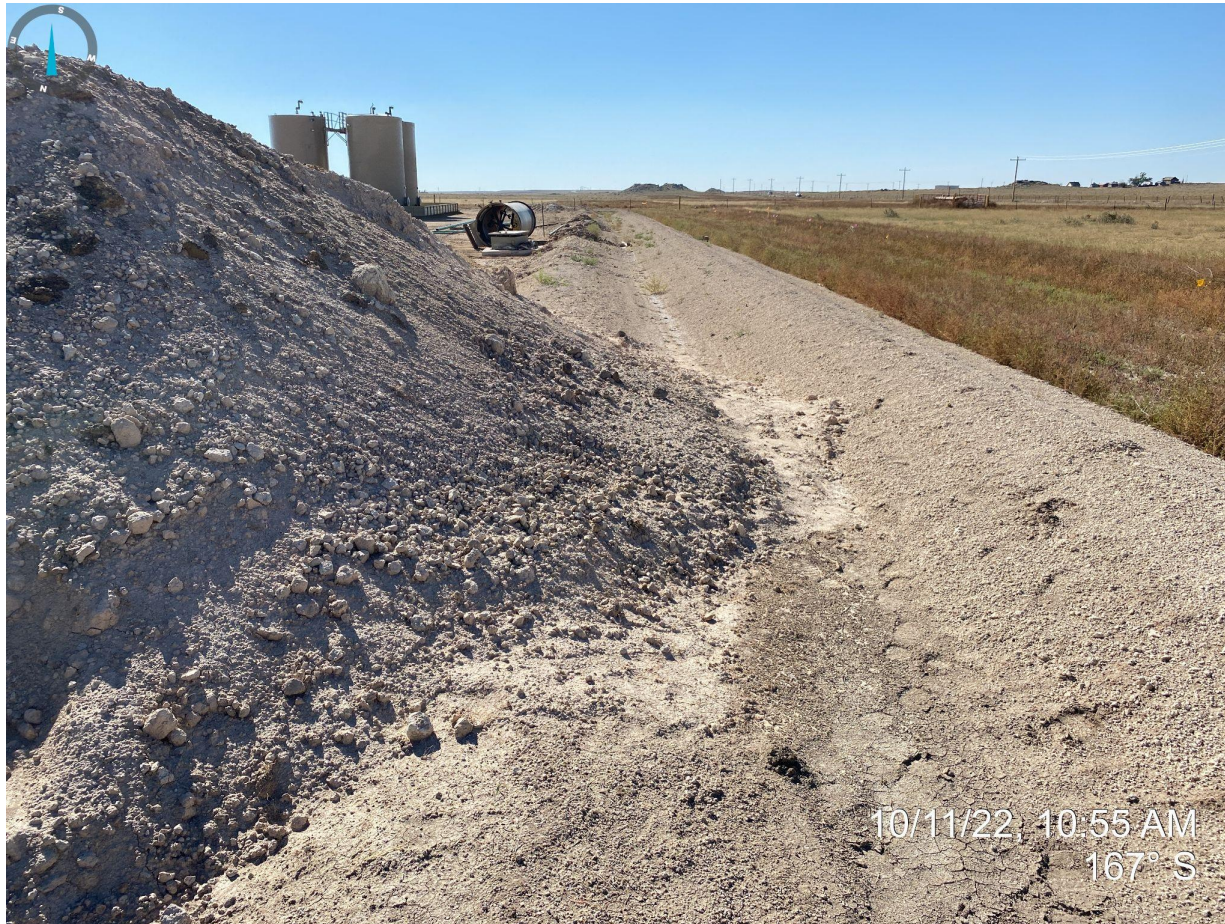
Photo 22. Taken from western portion of location, facing south. Photo depicts soil deposition in ditch and berm BMP.
