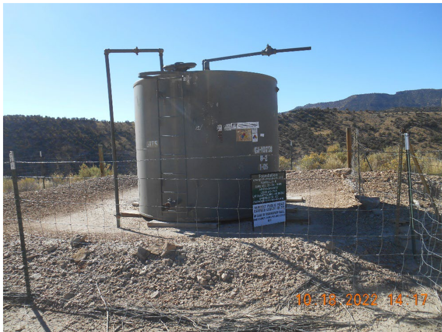
Condensate tank battery
