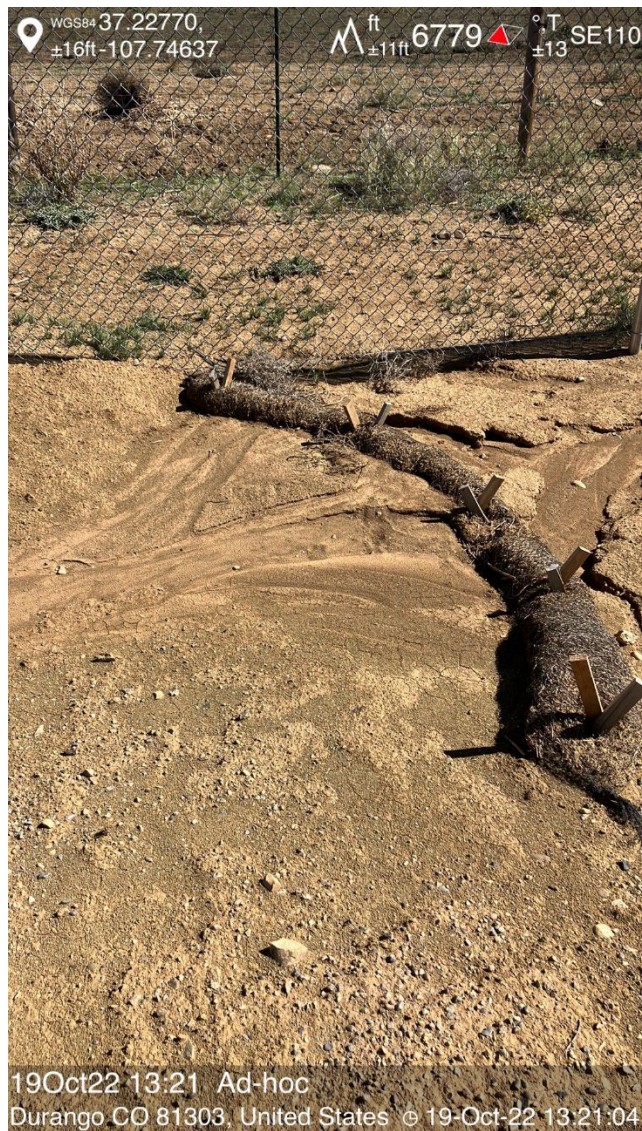
IMG 05 Waddle filled with sediment
