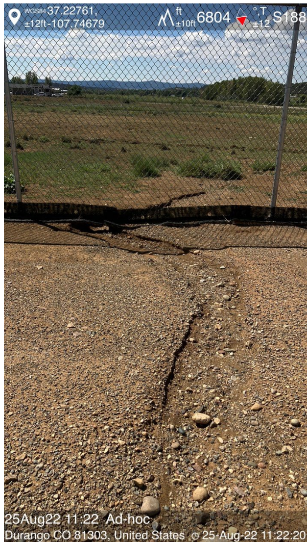
IMG 03 Erosion channel, 8/25/22
