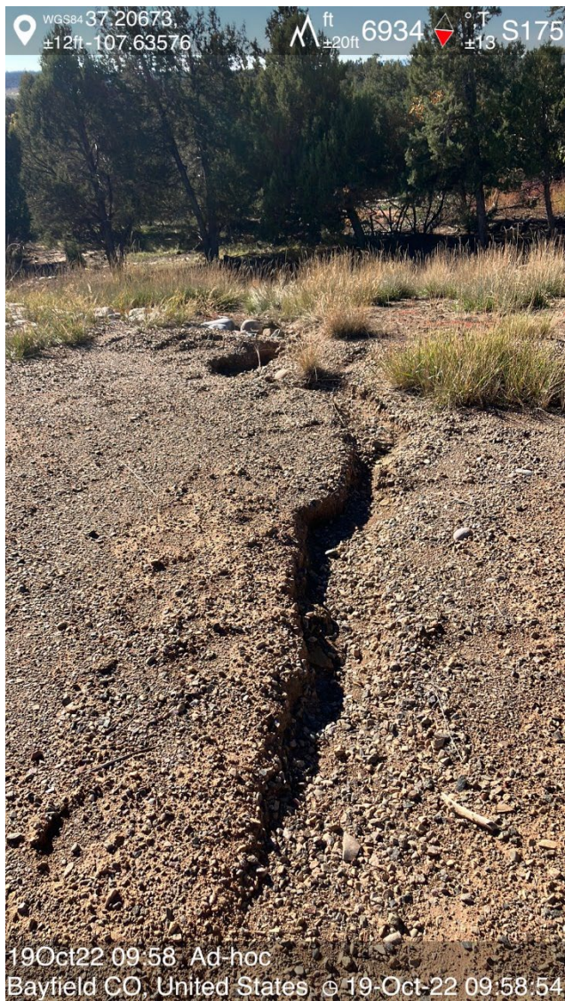
IMG 05 Erosion channel
