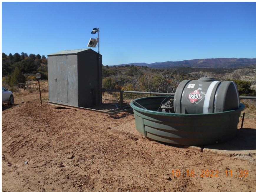
Meter housing. Secondary containment of chemicals
