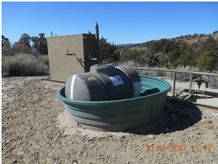
Separator and Secondary containment of chemicals
