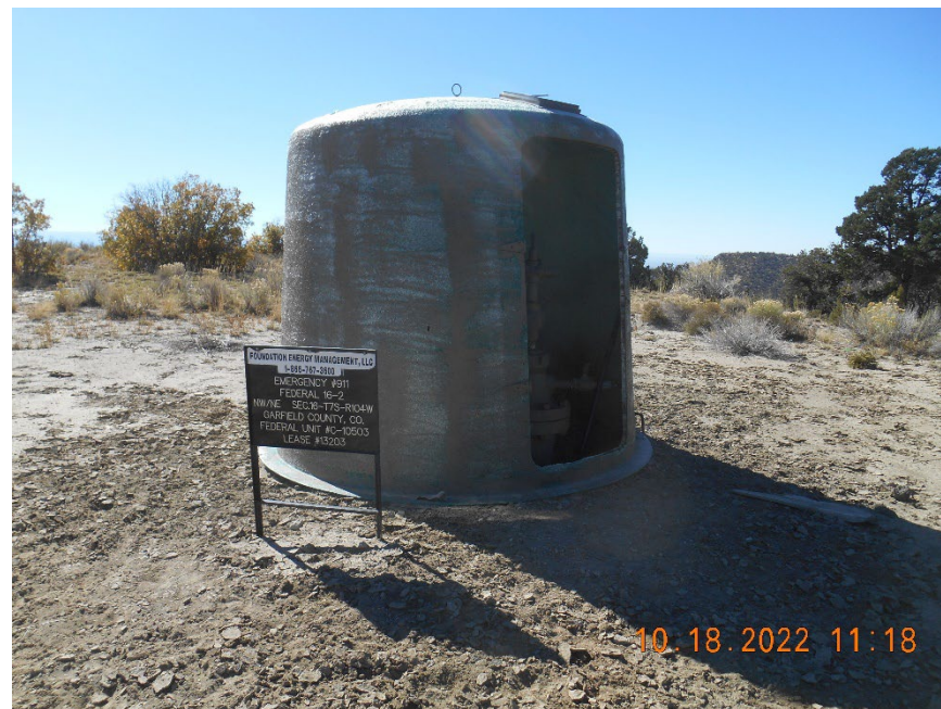
Wellhead inside fiberglass housing
