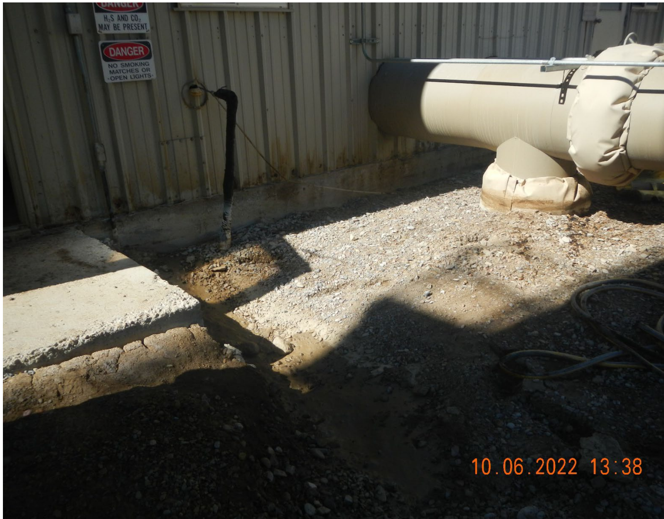
Photo #1 Area near spill origin. Note staining on pipe insulation.
