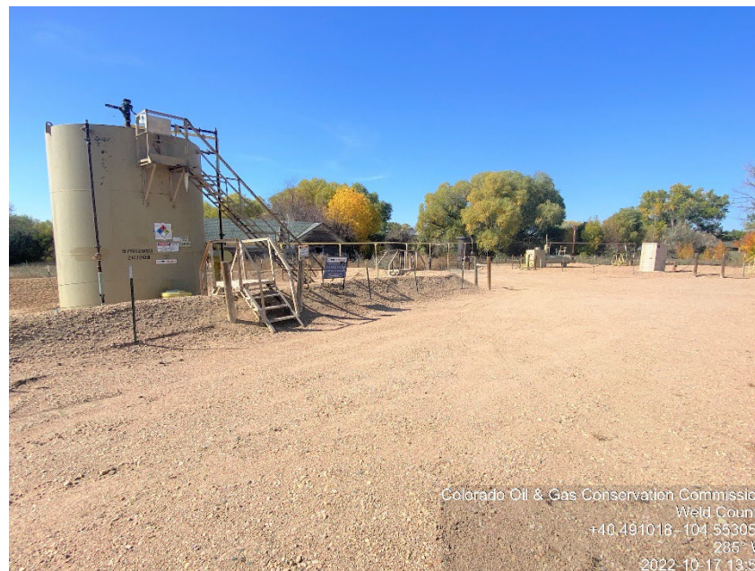
Photo #2 State 81 41-16 Tank Battery Battery site Inactive / Shut-down Equipment documented Fac. ID 466746 Formerly served: State 16C; Plugged & Abandoned | PA
