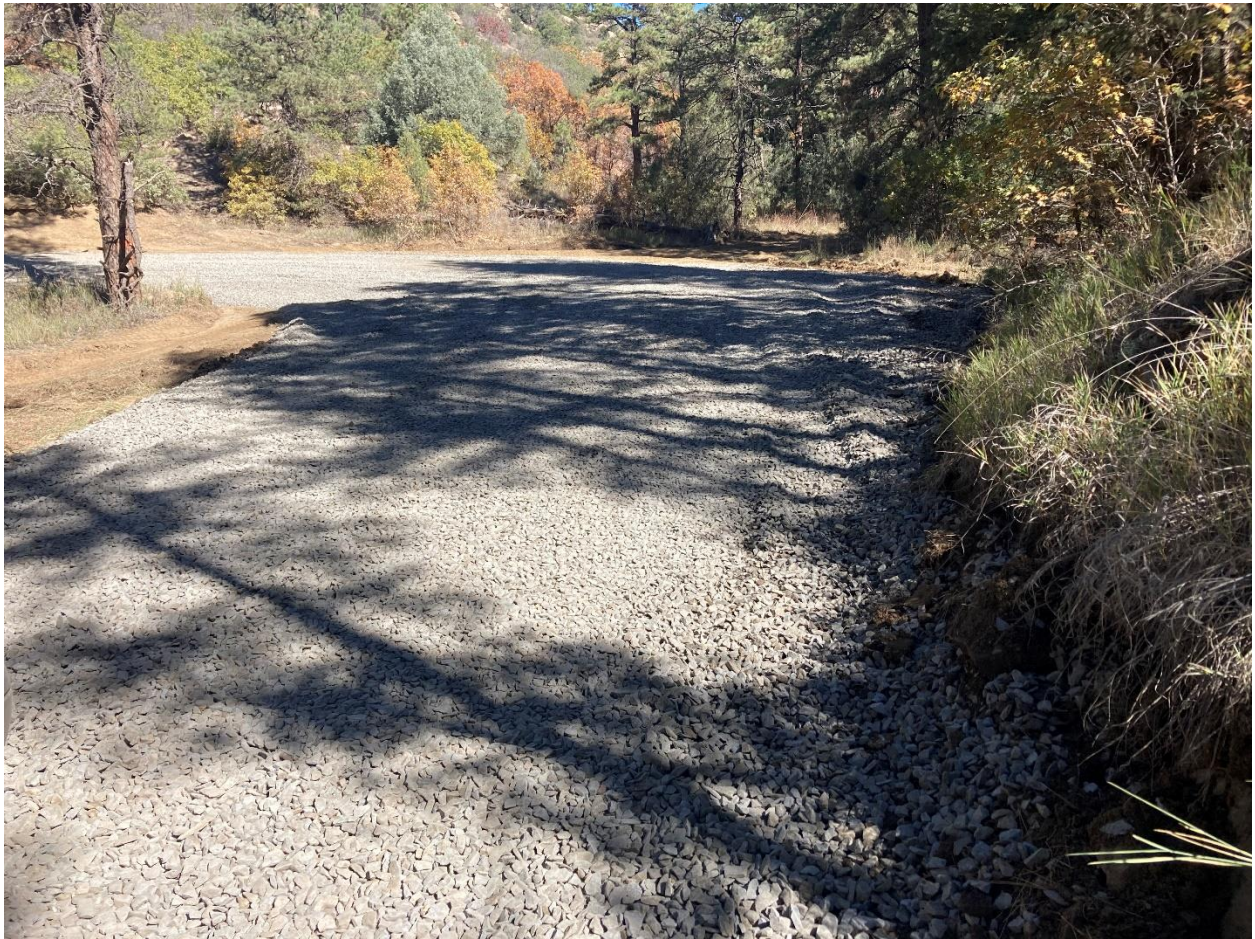
Additional stabilization provided installed and repaired required BMP's per Rule 1002.f.(2)C
