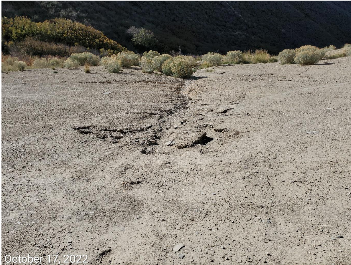
Photo 8: Photos 8-11 taken from the southwestern production areas of the Location. Photos show stormwater discharge point from the pad has not been constructed with a properly engineered outlet; stormwater runoff has resulted in degradation at the outlet, with erosion progressing into the working pad area.
