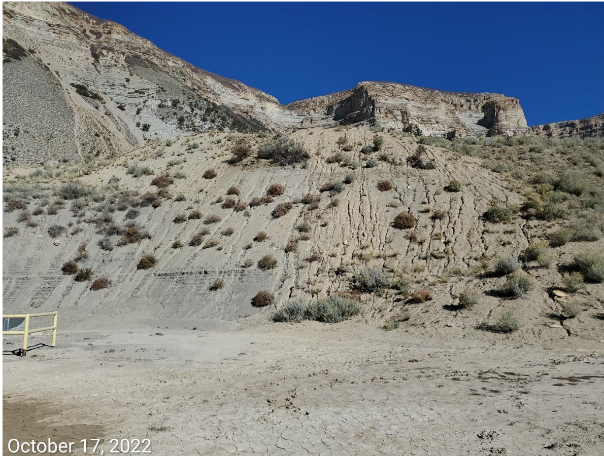
Photo 2: Photos 2-7 show erosion degradation and sediment deposition (yellow arrow) due to missing or insufficient stormwater and erosion control BMPs at the cut slopes of the Location
