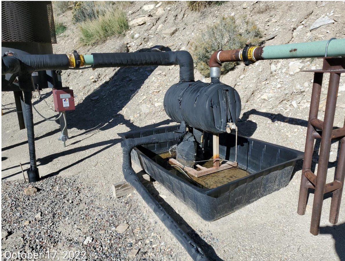
Photo 14: Secondary containment missing wildlife protection BMPs.
