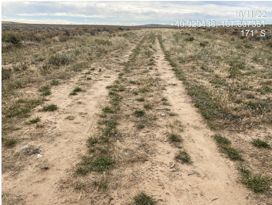
Photo 1. Photo taken from the Location entrance shows the access road is bare and compacted in tracks. Vehicles are utilizing the road, potentially compromising revegetation.
