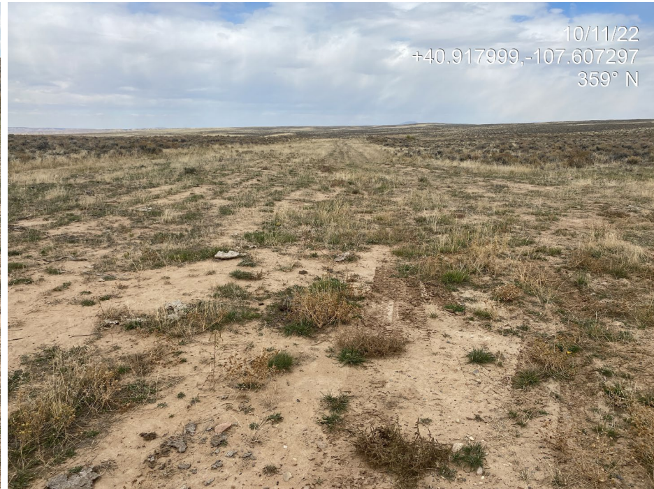
Photo 2. Photo taken to the south shows the start of the access road. Portions of the road are revegetated, however, perennial cover is not uniform. Bare ground and annual weeds are common and vehicles are utilizing the road causing compaction and potentially compromising revegetation.
