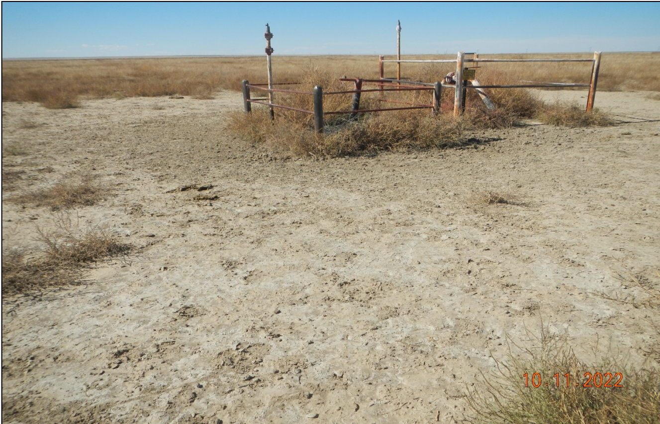
Photo 3. There are pipe risers associated with the former well site that have not been removed. Previous corrective action was not completed.
