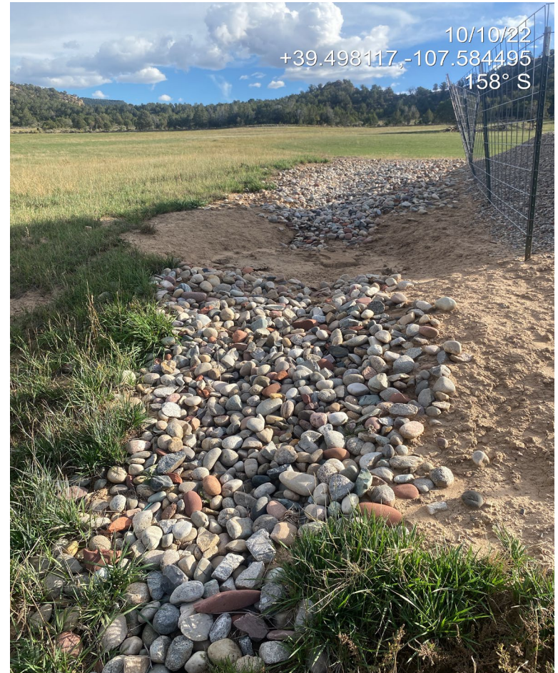
Photo 6. Photo shows a stormwater BMP at the northeast of the Location. The structure is installed with smooth river rock and lacks a geotextile liner. No degradation was observed.
