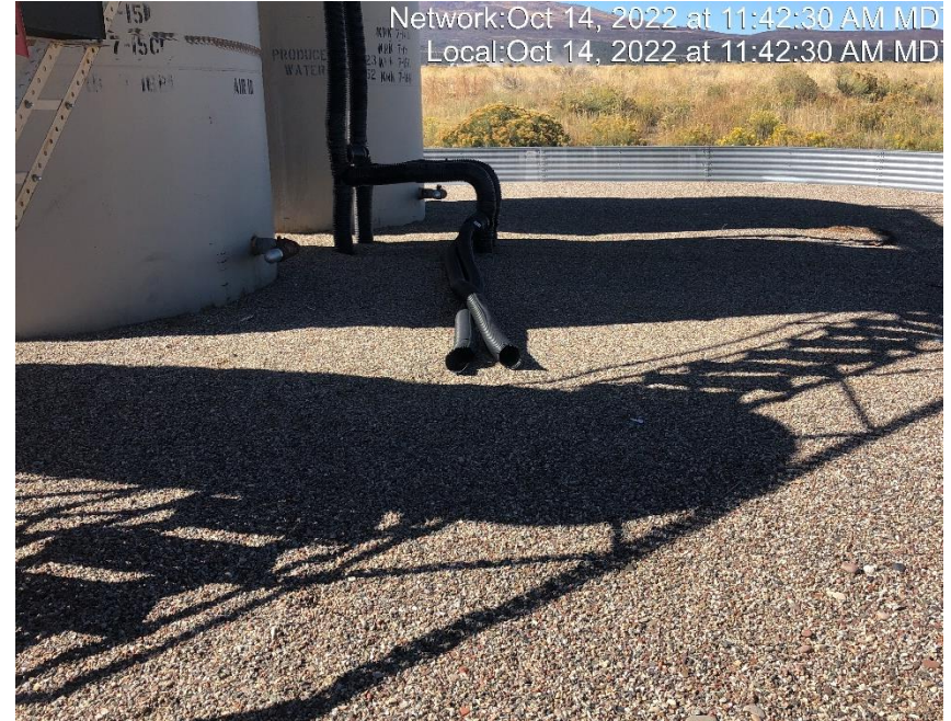
Photo #8083 Flow line heating insulation open ended.
