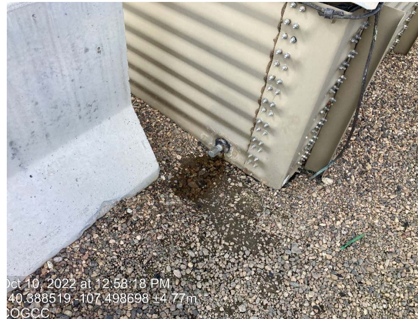
Plug on tank battery containment is actively leaking
