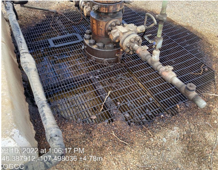
Staining and cellar is full of fluid possible crude
