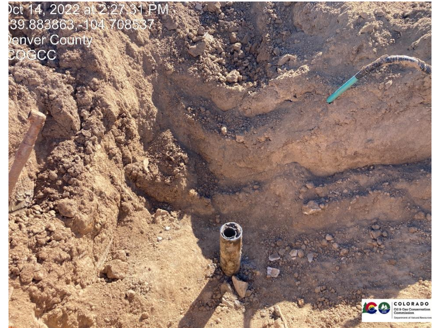
Pic 2 casing, wellhead has been cut.
