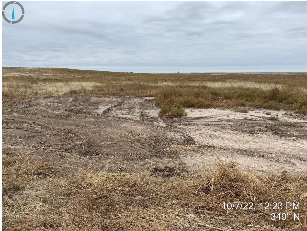
Photo 1. Taken from meter location, facing north. Photo illustrates that all oil and gas equipment has been removed from the location and that it has not been reclaimed (e.g. not contoured, graded, revegetated).
