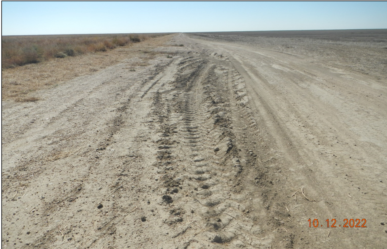
Photo 1. Facing south along the access road. The road is not maintained and vehicle are driving around the rutted area causing widening of the road.
