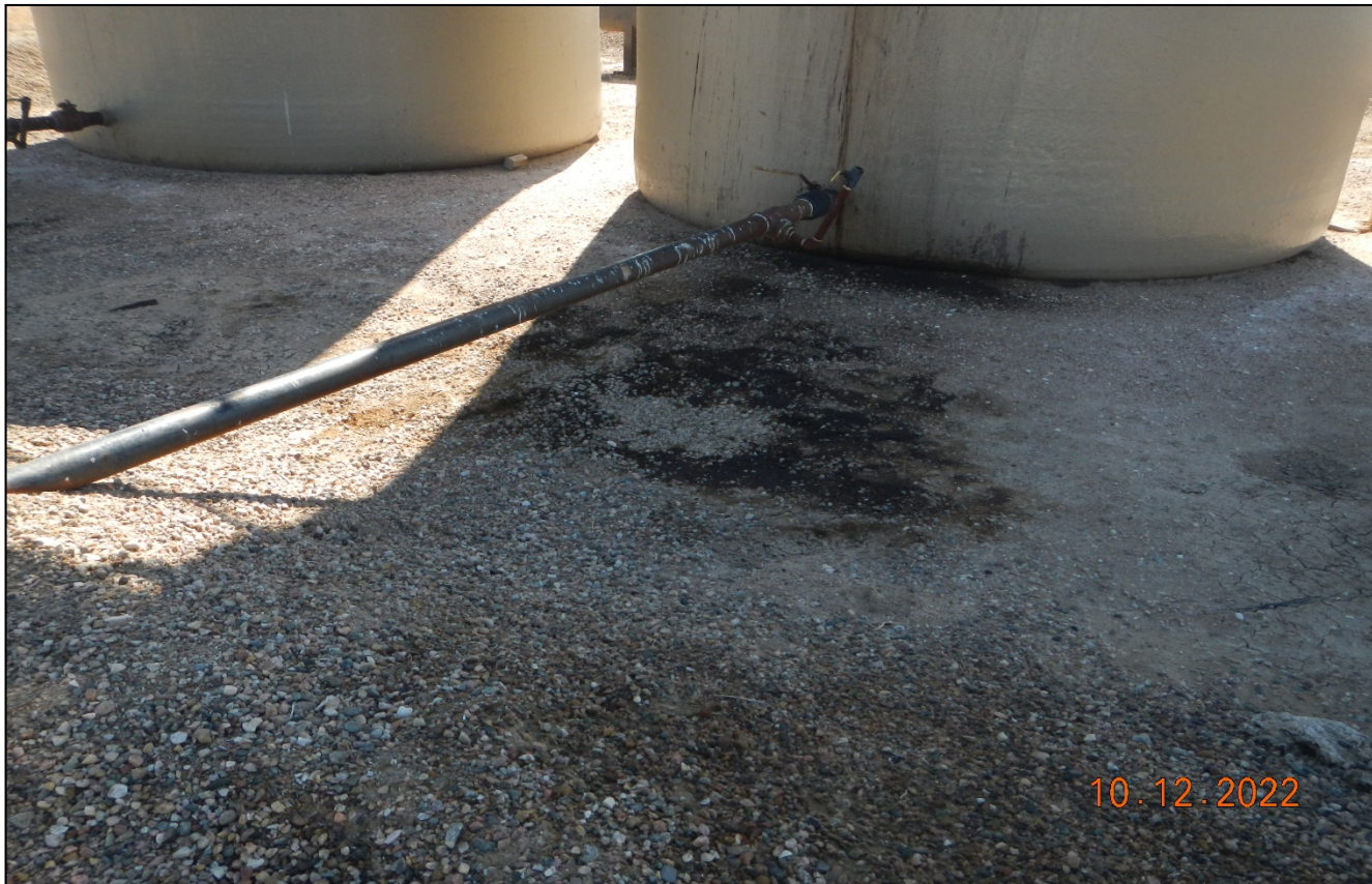
Photo 4. There are oil stained soils inside the containment that needs to be cleaned up.
