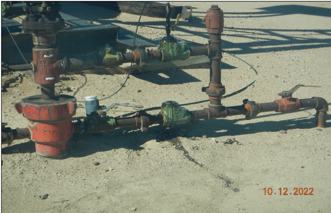
Photo 7. There was a dripping leak occurring at the pipe fittings.
