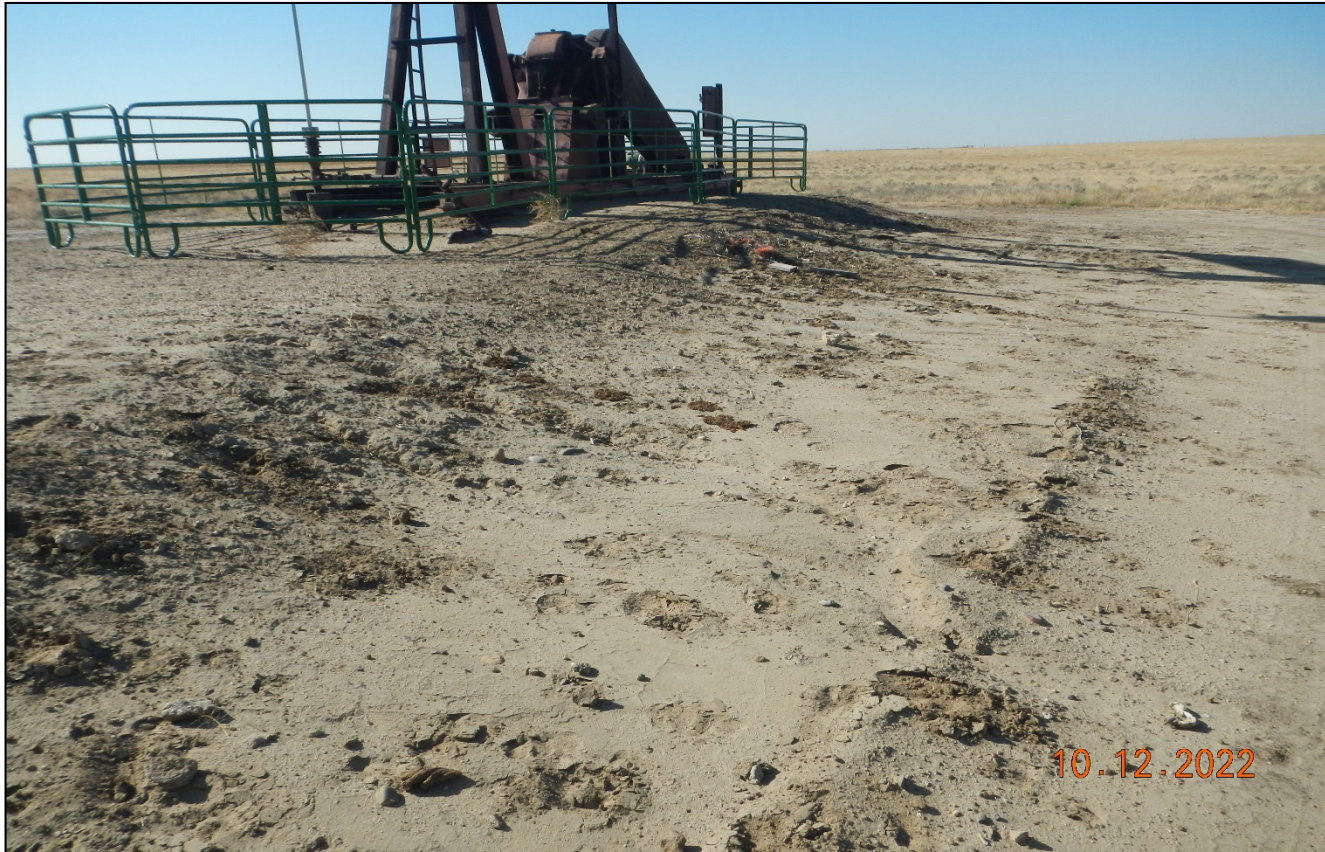
Photo 4. Facing toward the pumpjack. There is stormwater runoff transporting sediment offsite. Previous corrective action not completed to install BMP's.
