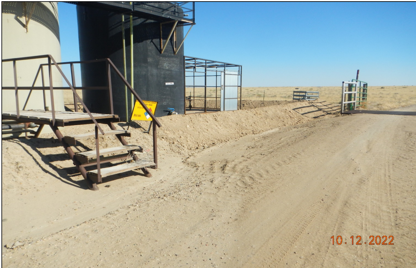
Photo 3. A secondary containment berm has been installed around the tank battery. The berm still needs to be compacted.
