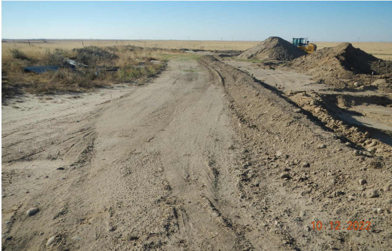
Photo 3. Facing south toward the east side of the tank battery location. A berm was installed around the perimeter of the soil piles. Berms are not compacted and may not withstand heavy precipitation.
