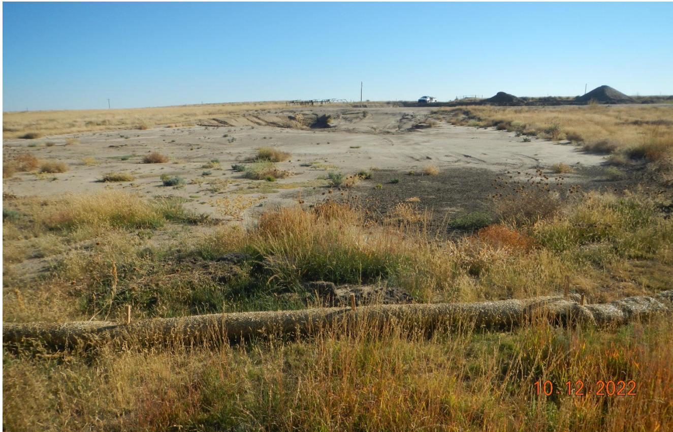
Photo 7. Facing northeast at the down gradient side of the spill area. Straw wattles have been installed along the edge of the disturbance.
