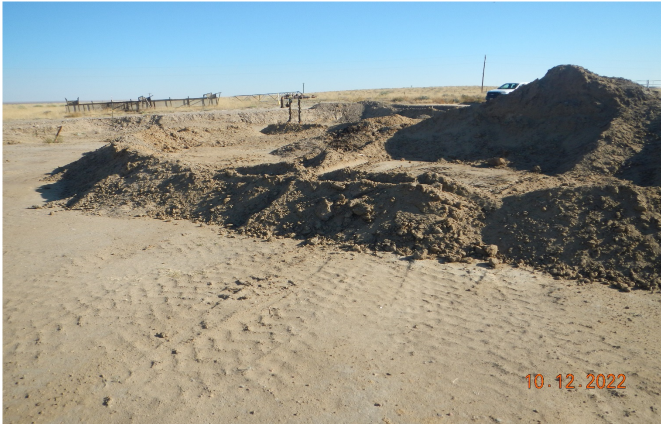
Photo 4. The berms around the soil piles have been constructed larger but were not compacted. Also, no liner was observed under the contaminated soils. Contaminated soils should be removed and properly disposed.
