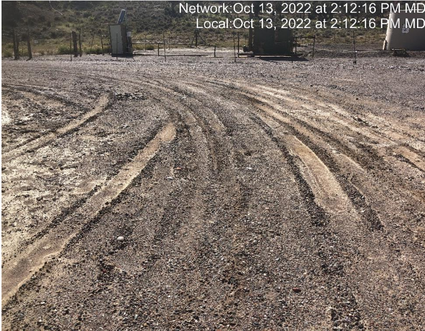
Photo #8061 Location lacks stabilization.
