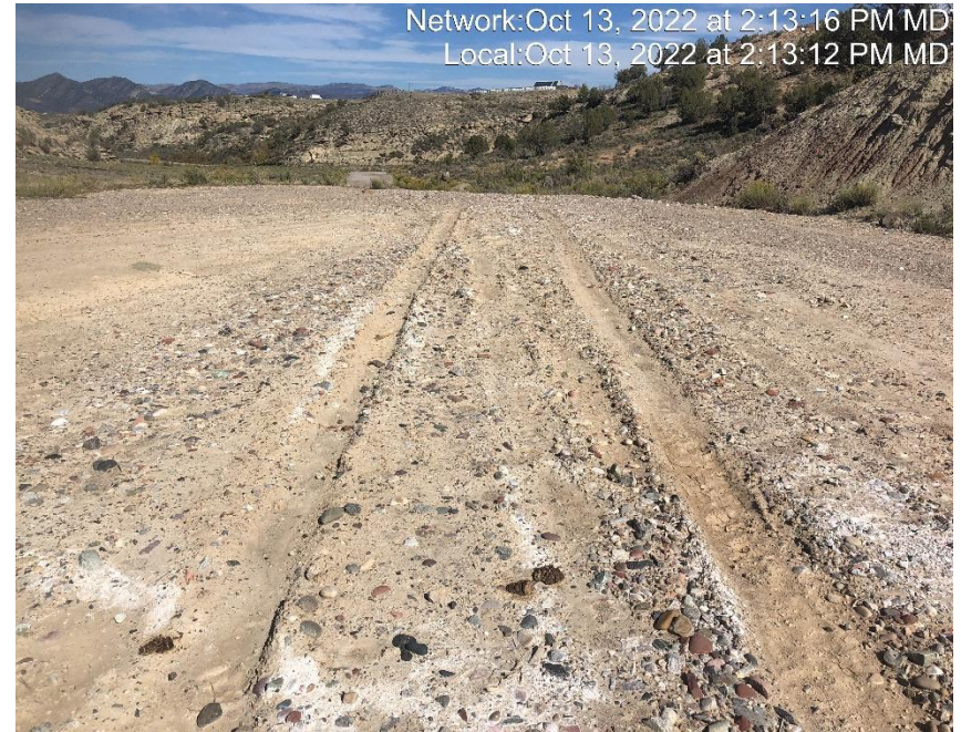
Photo #8064 Insufficient tracking BMP at entrance to location.
