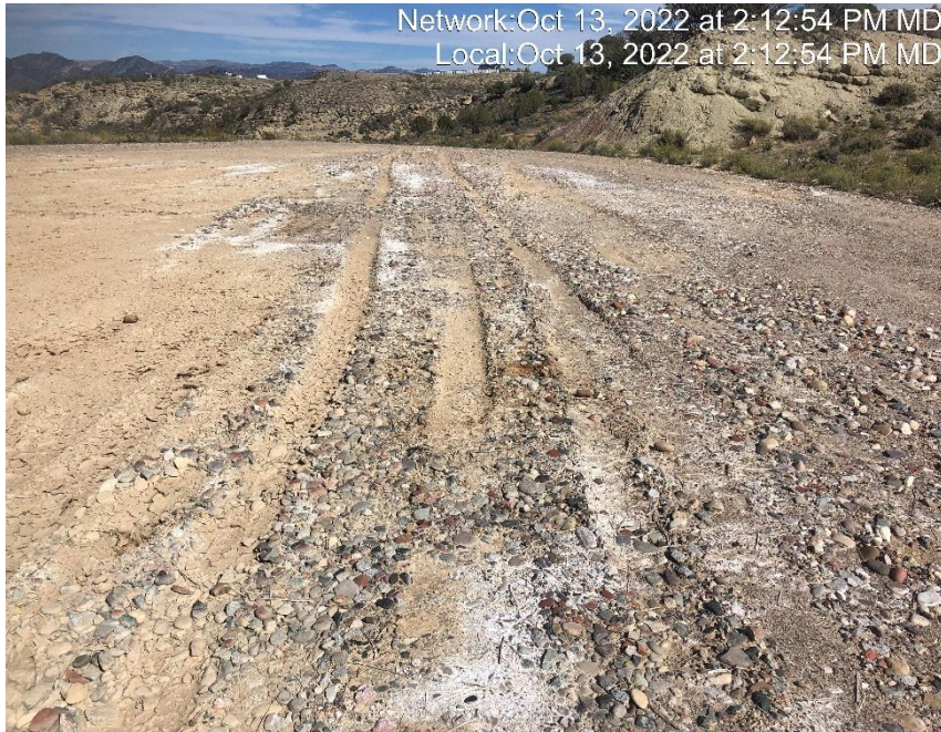
Photo #8063 Location lacks stabilization.
