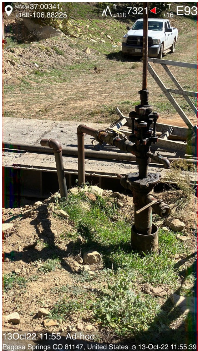
IMG 03 Wellhead
