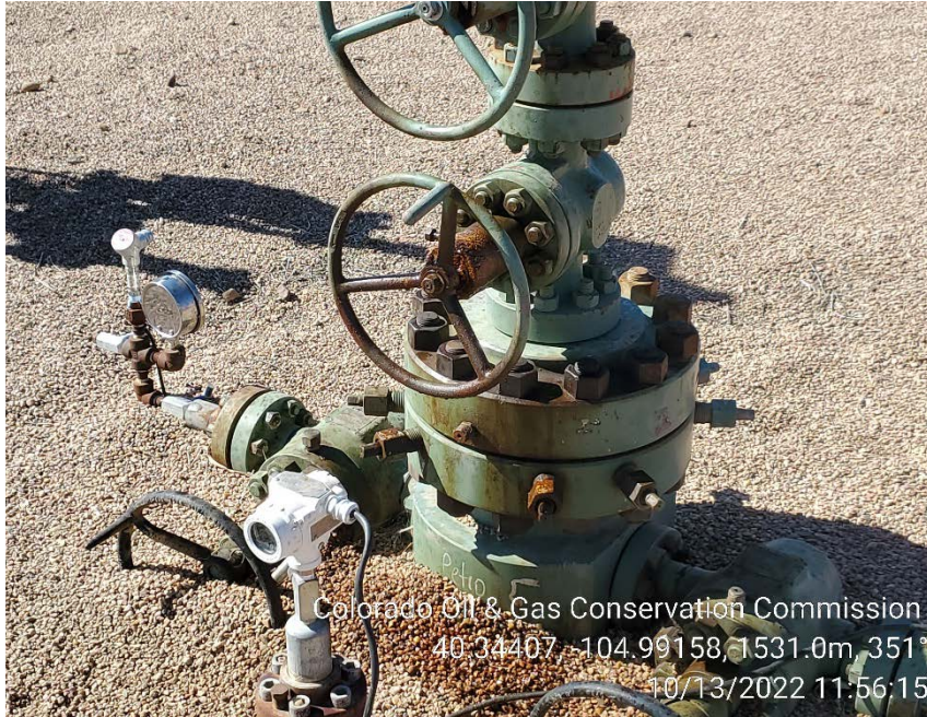
Master valve leak and stained soil
