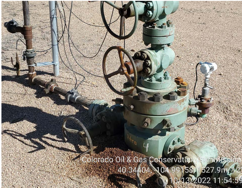
Master valve leak and stained soil
