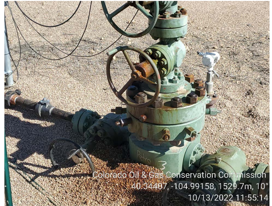
Master valve leak and stained soil
