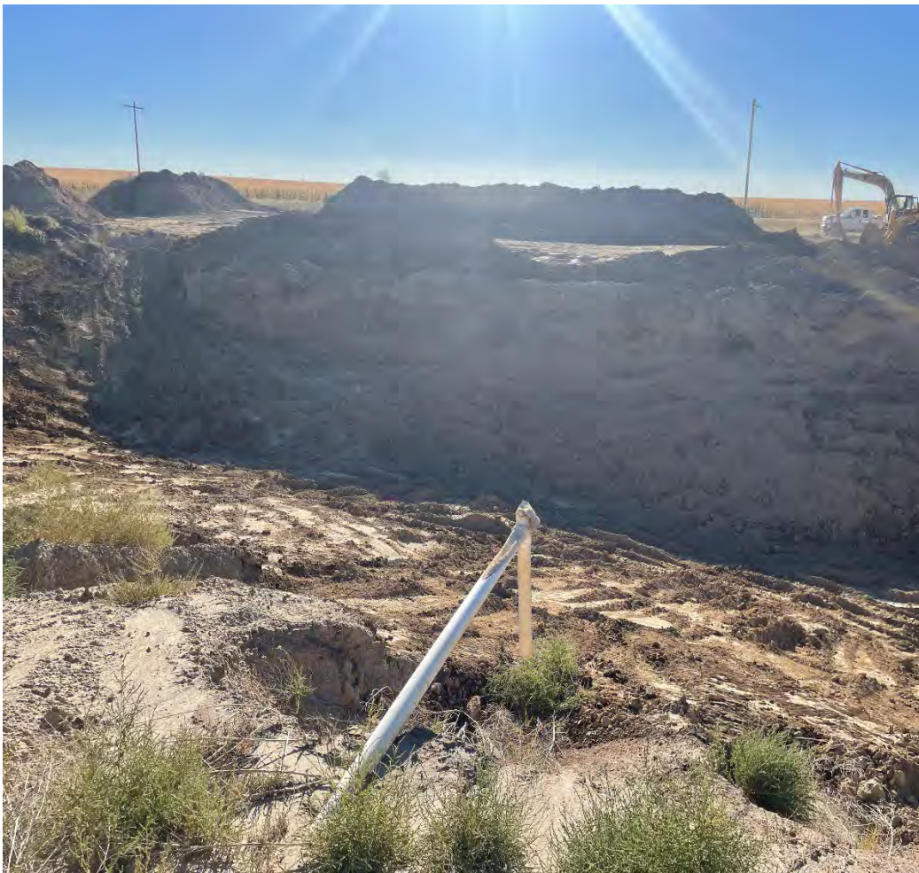
West Pit following removal of impacted soils 9/29/2022
