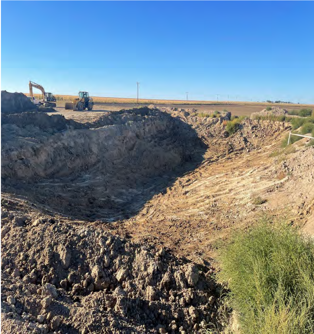
West Pit following removal of impacted soils 9/29/2022
