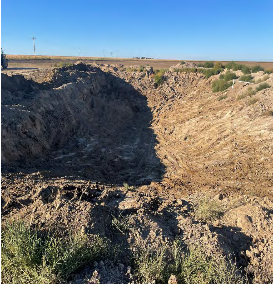
West Pit following removal of impacted soils 9/29/2022
