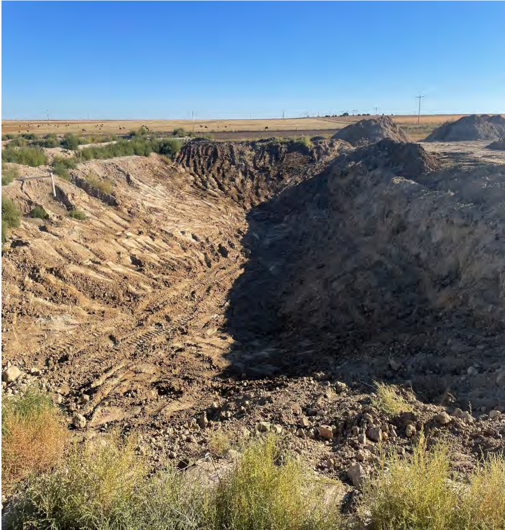
West Pit following removal of impacted soils 9/29/2022
