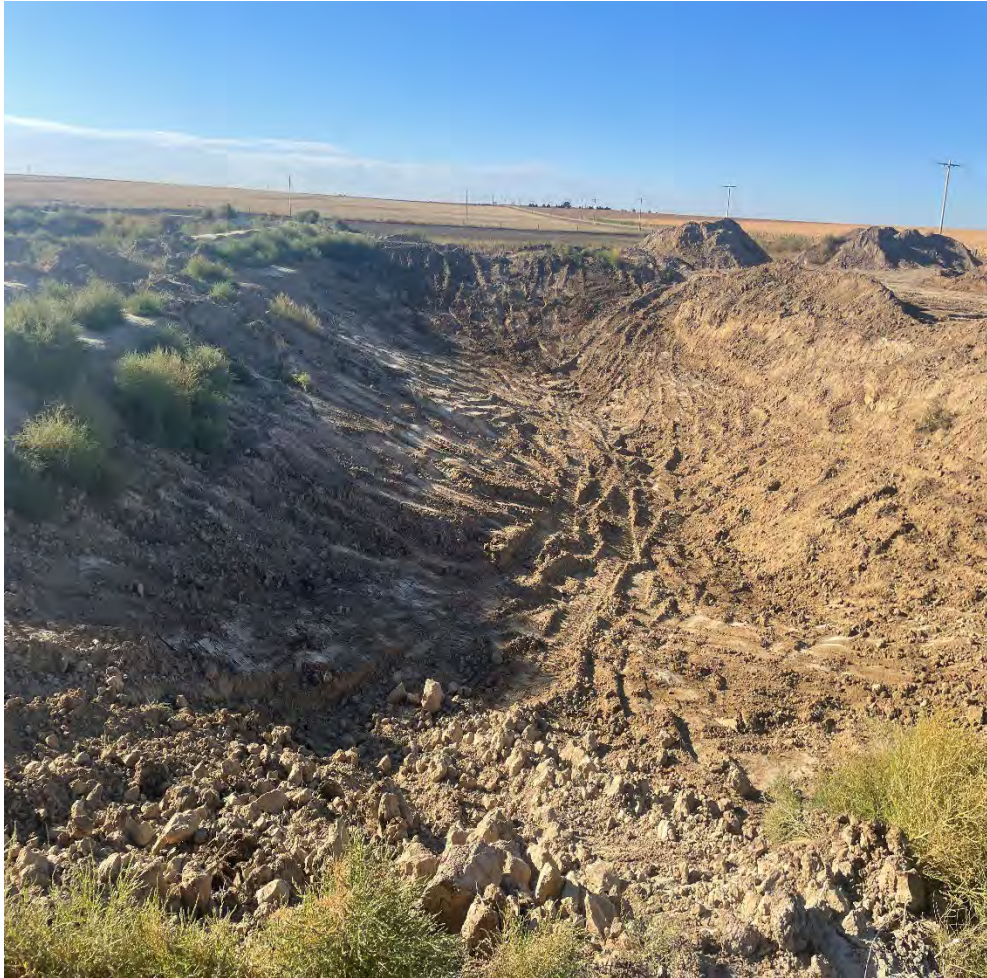
West Pit following removal of impacted soils 9/29/2022
