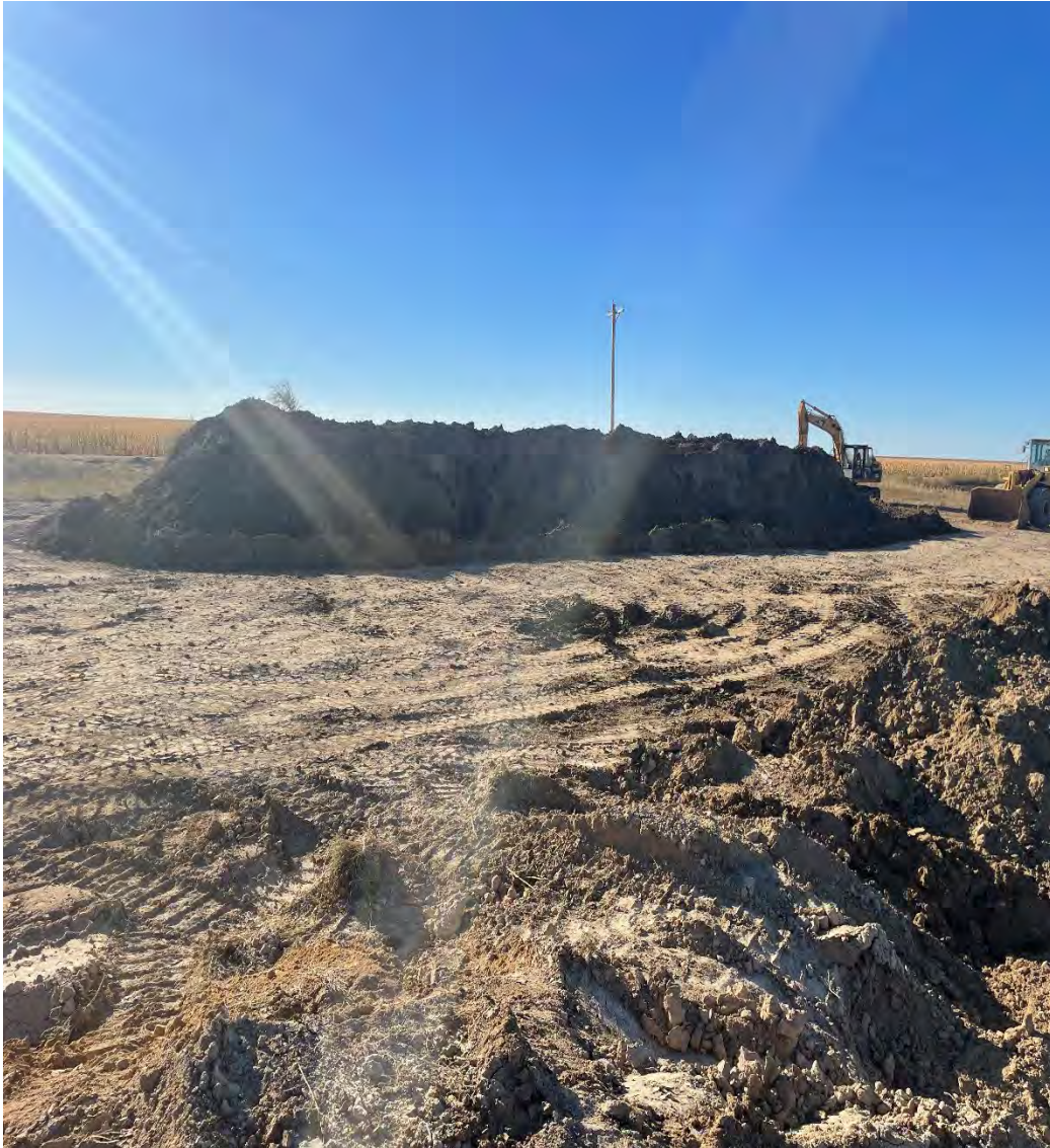
West Pit stockpiled soils following removal of impacted soils 9/29/2022
