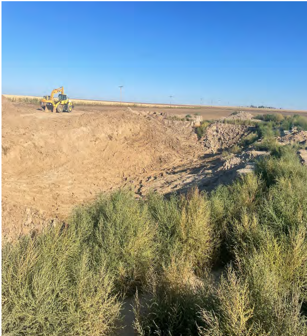
West Pit following removal of impacted soils 9/29/2022
