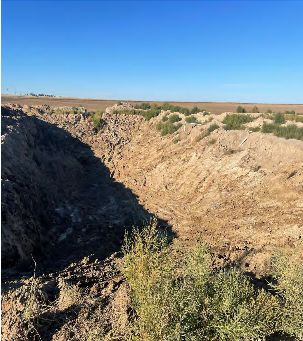
West Pit following removal of impacted soils 9/29/2022
