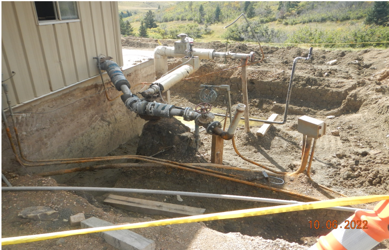
Photo 3. Facing where tank was located. Impacted soil were excavated from this area.
